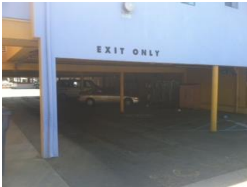
View of parking area under 1123 Fremont Boulevard
