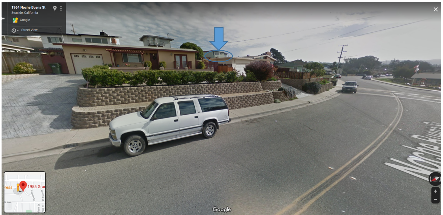
View of 1955 Grandview and new deck coming from the north on Noche Buena (view from north).
