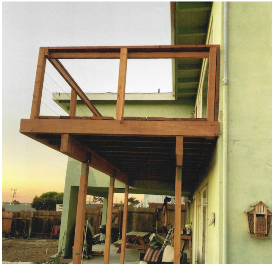
View from the east of new 160 sf redwood deck.
