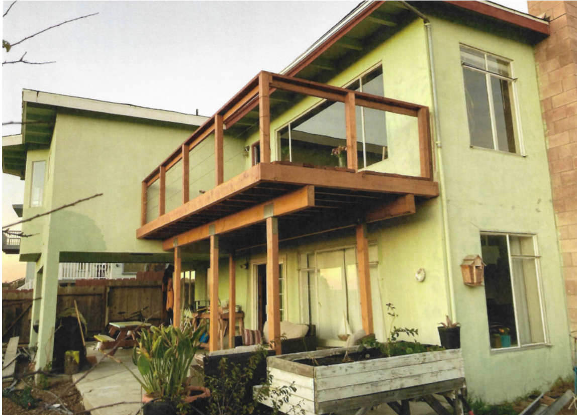
Photo of new 160 sf redwood deck.
