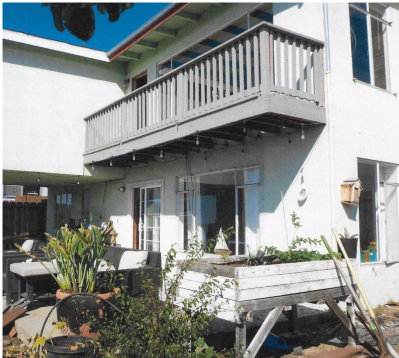
Photo of the old 80 sf deck which was demolished.
