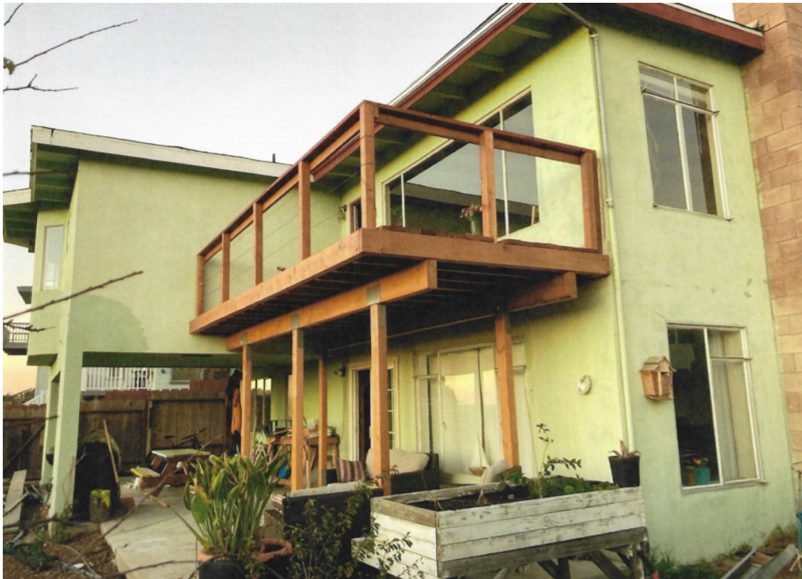
Photo of new 160 sf redwood deck.
