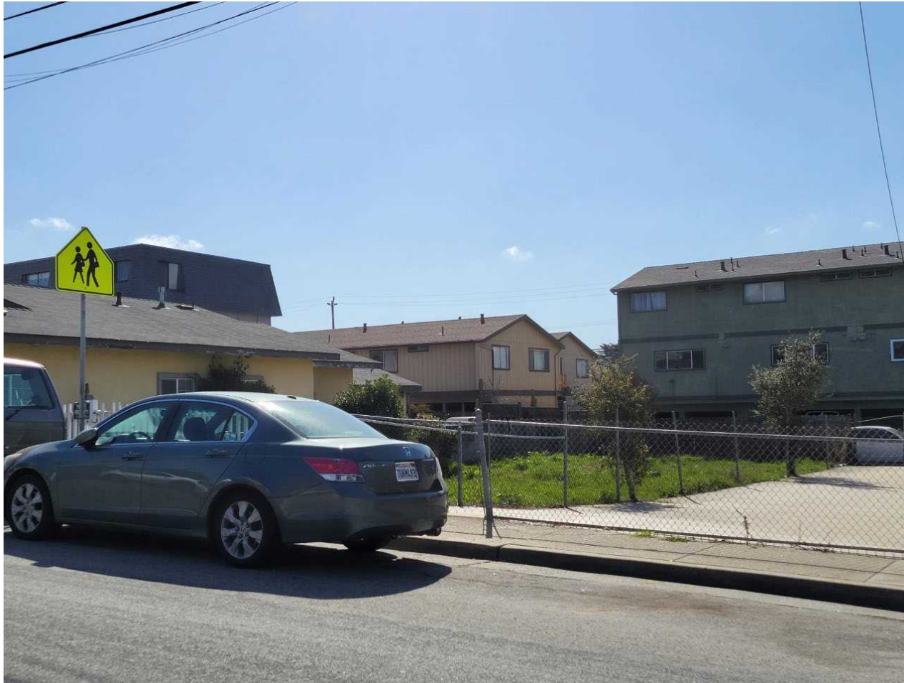
Surrounding multi-story, multifamily housing.
