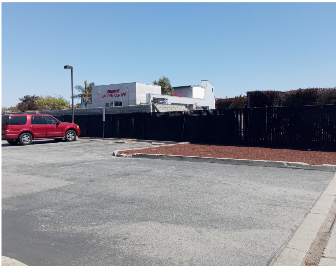
View of existing CMU wall from Dollar Tree parking lot looking east.
