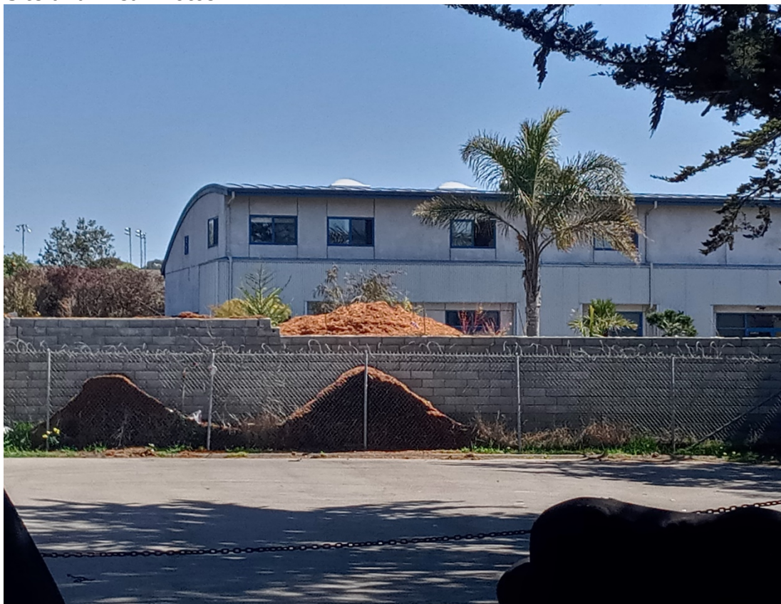
View of existing CMU wall from Goodwill along Fremont looking east.
