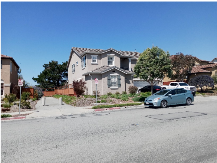
Property to north with (e) front balcony.
