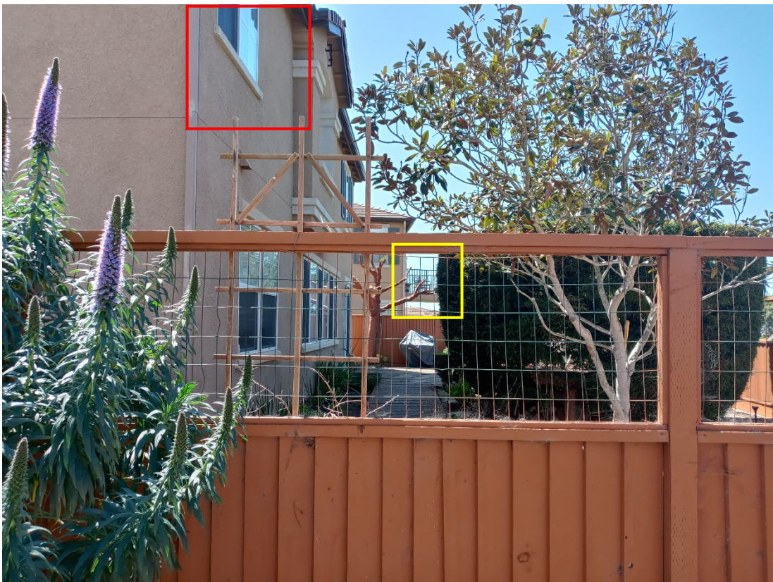
View from public ROW between 4456 and 4460 Ocean Heights Court looking south. Neighbors existing deck is visible (yellow) and the proposed location of the new deck is marked in red.
