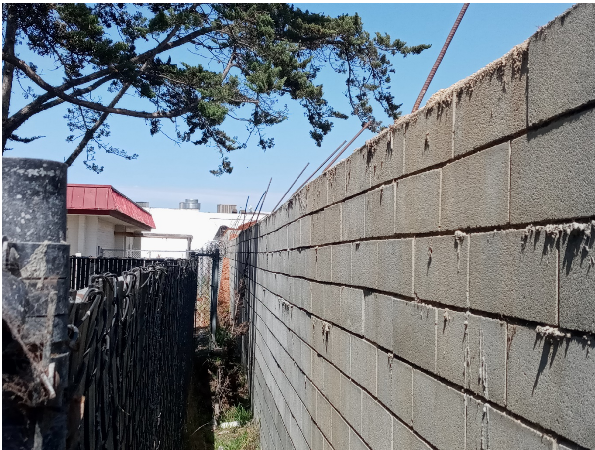
View of CMU wall looking along western property line (north)
