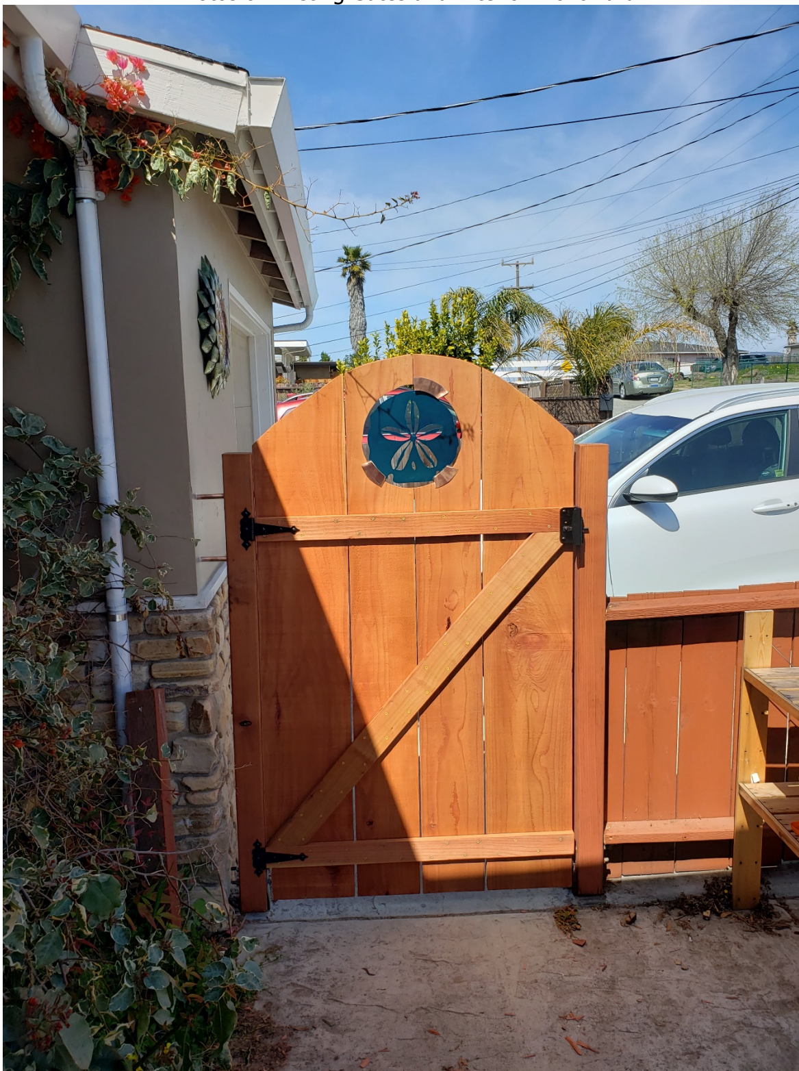
Photo of existing, newly constructed and installed, front entry gate.
