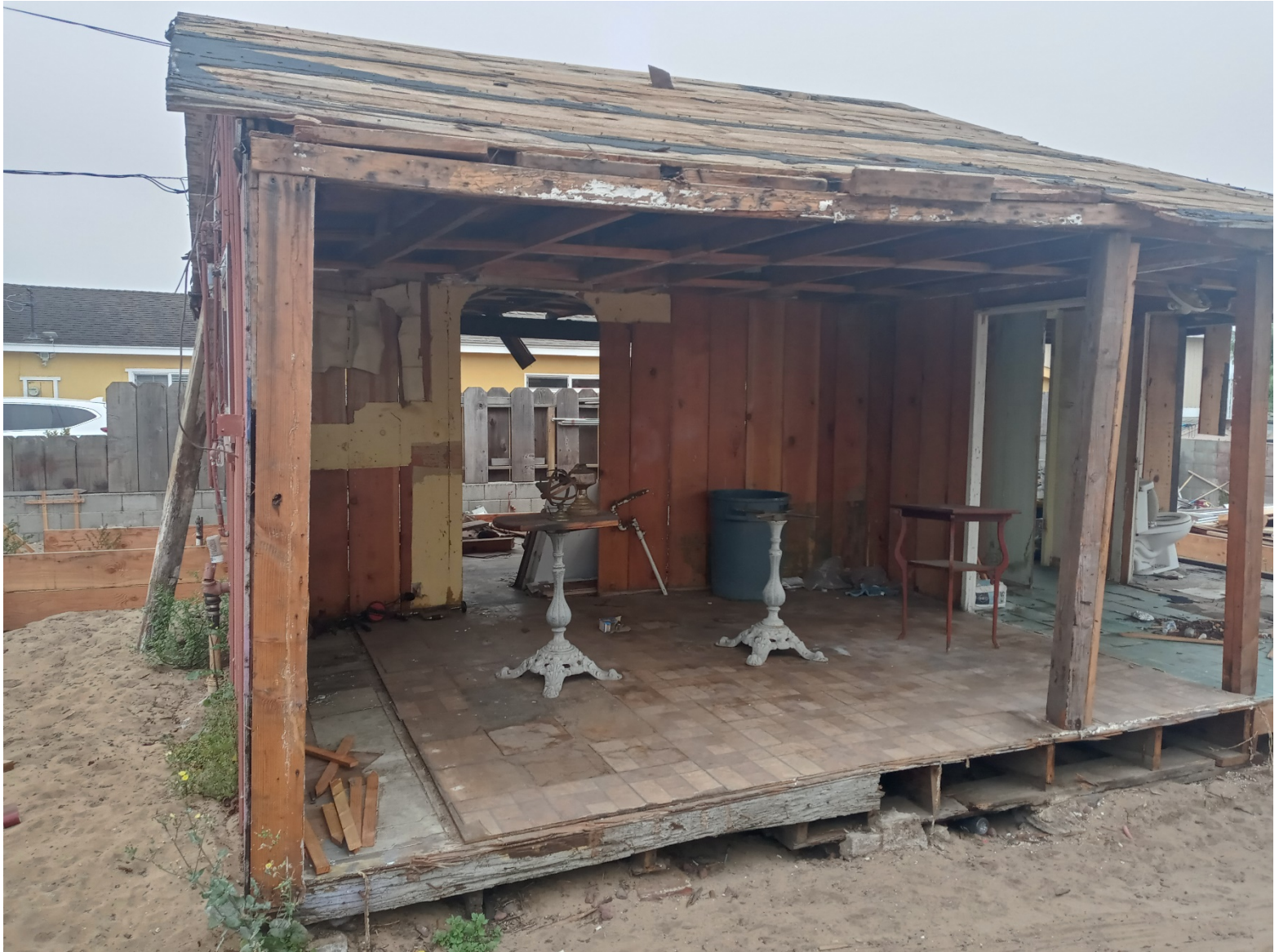
Existing house being demolished.
