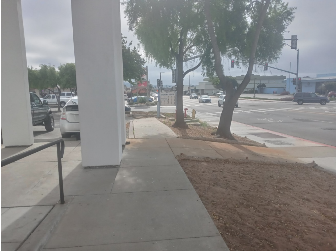
View from north side of building looking west towards intersection of Terrace + Broadway.
