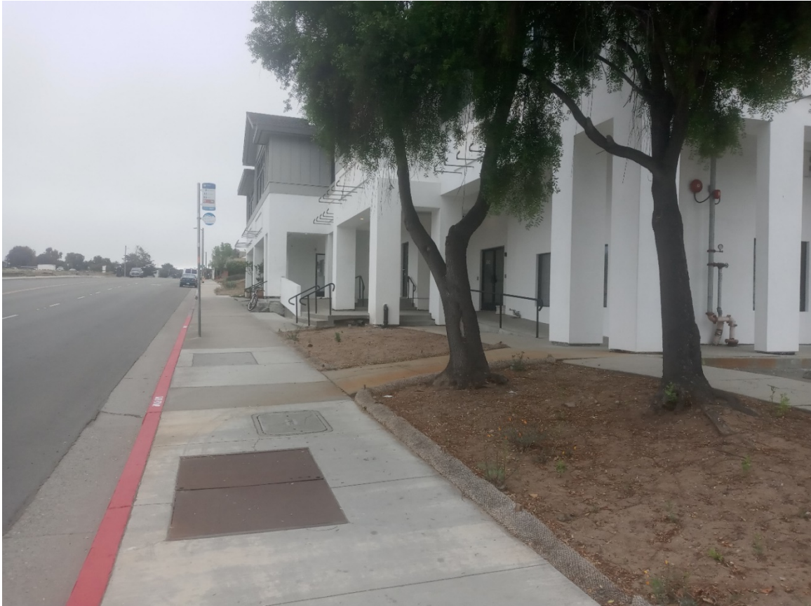
Looking east from corner of Terrace and Broadway.
