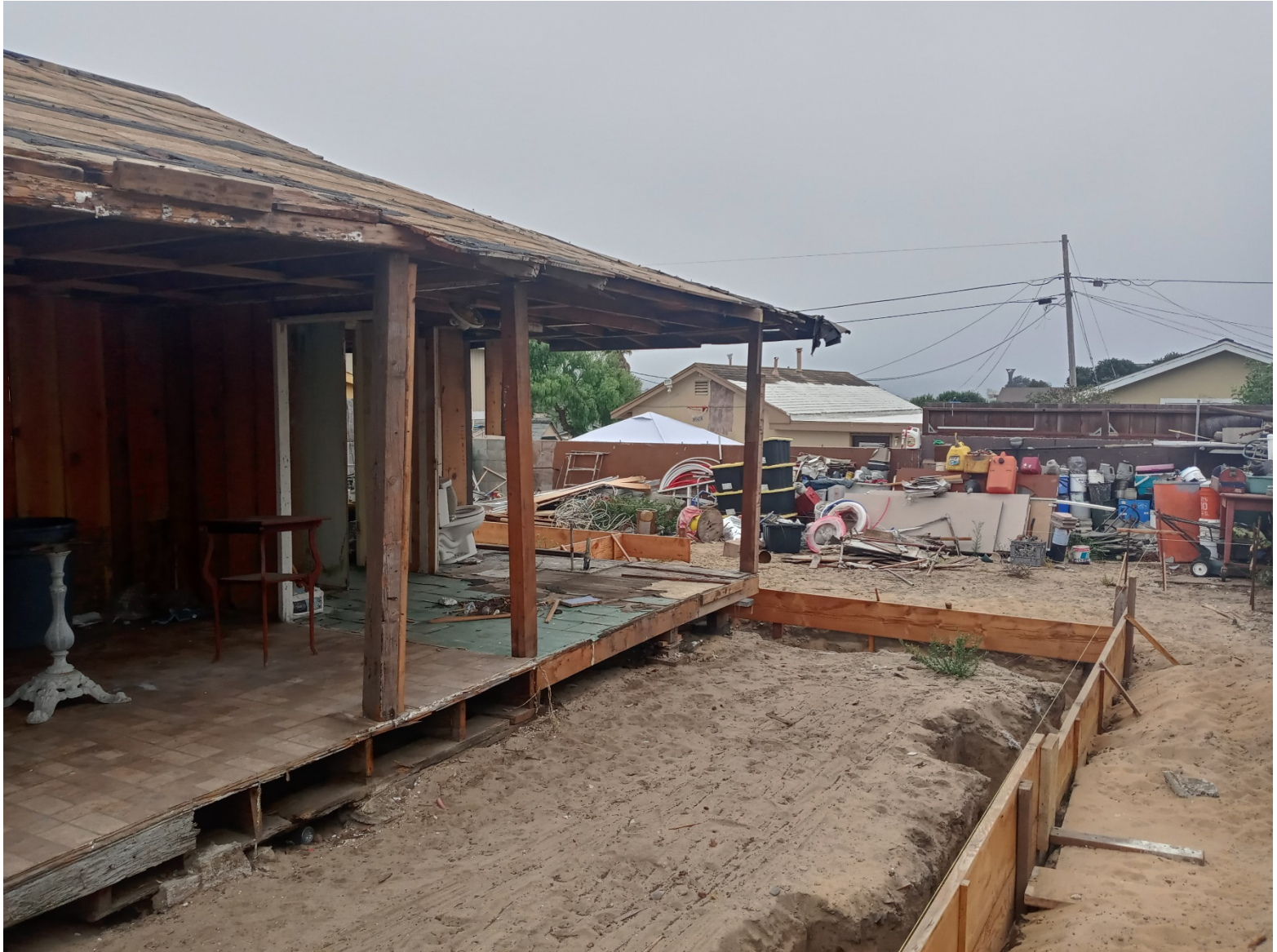
Existing home partially demolished.
