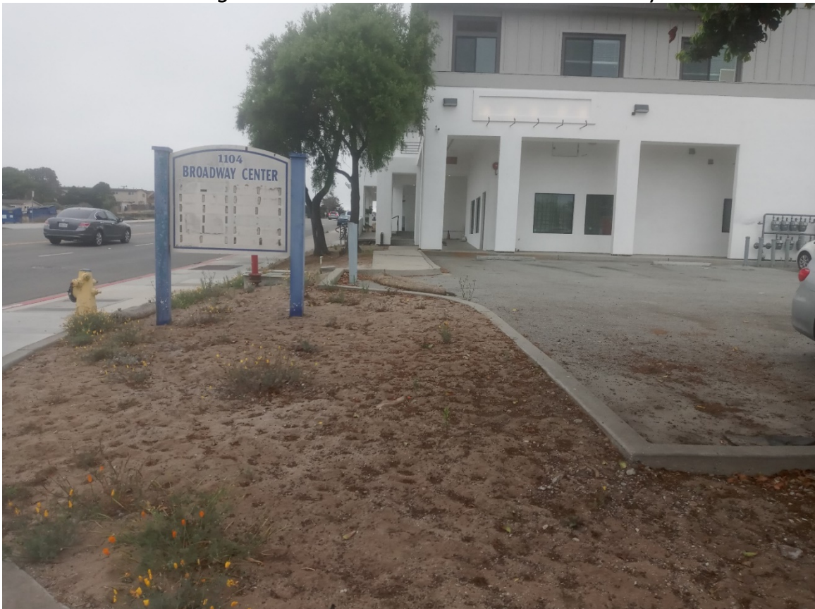
Looking east from Terrace Street.
