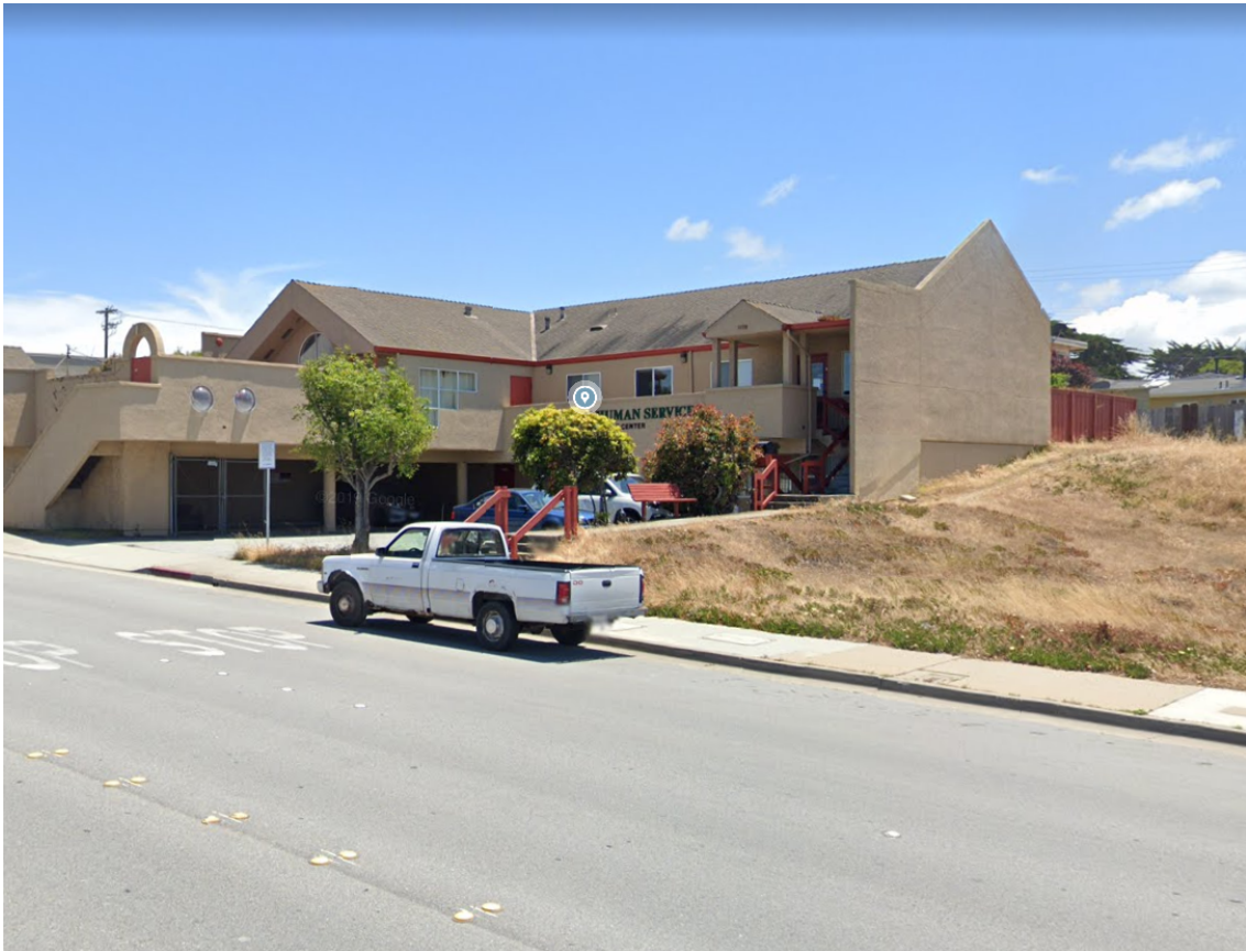
Property east of project site with no on site fencing along frontages.
