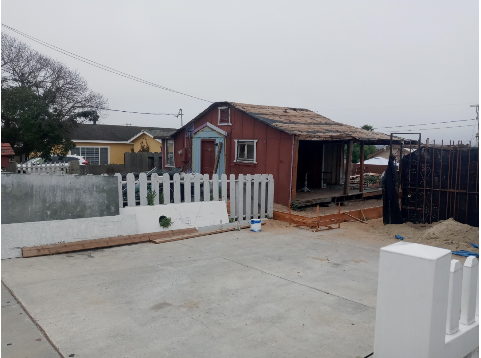
Existing house in process of being demolished.
