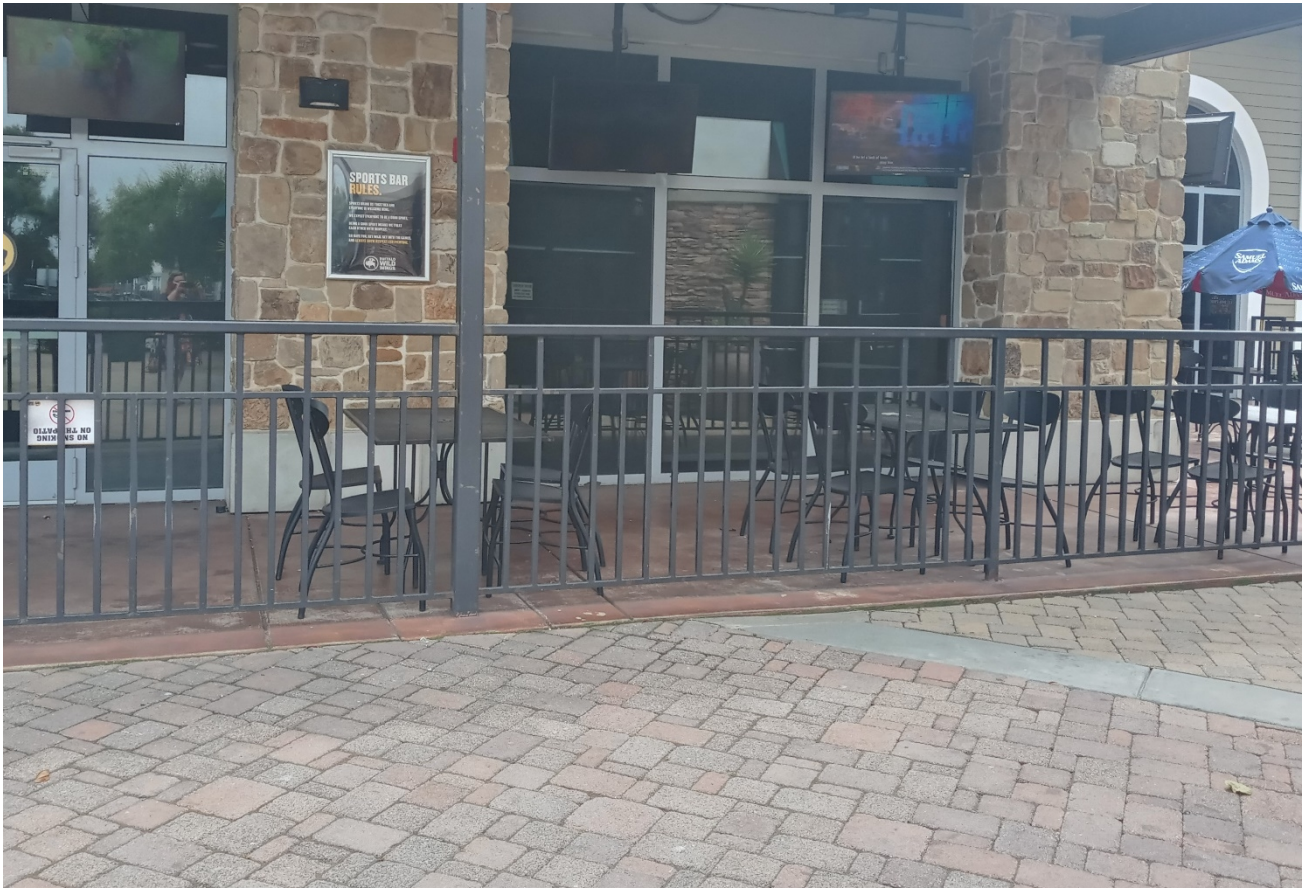
Fencing of neighboring outdoor dining area (Buffalo Wild Wings), applicant proposes to use same black metal fencing to match. [South]
