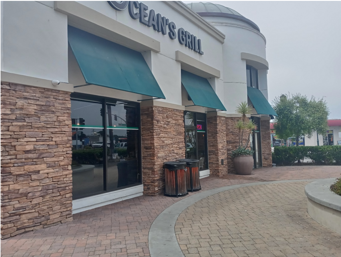
Current main entrance. [North]
