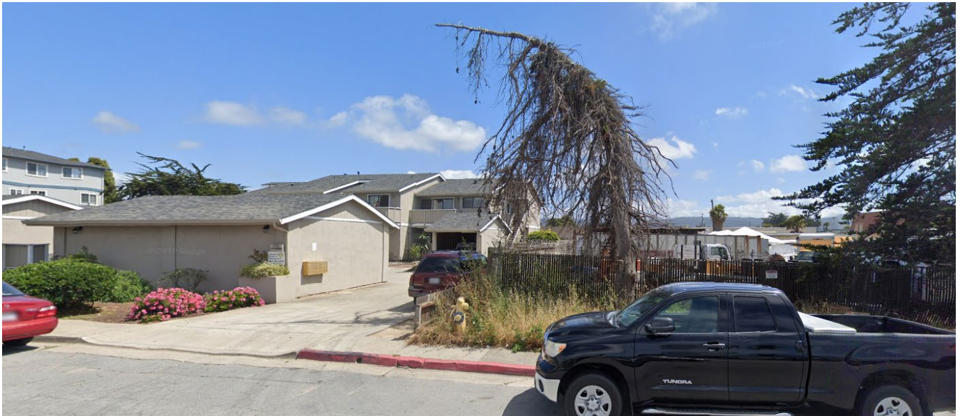
Properties immediately south (across San Pablo). Commercial on right, multi-family residential on left.
