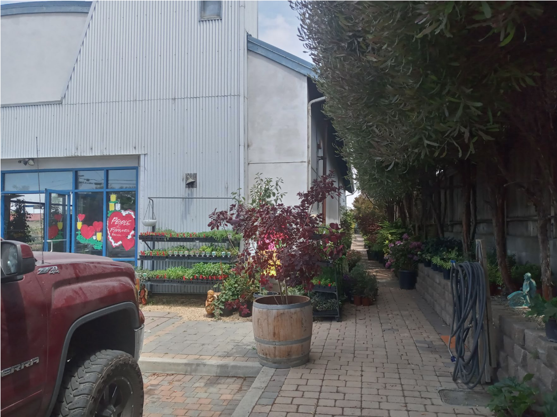
View along eastern property line, no exterior changes proposed to this frontage except installation of 1 egress window for one of the three bedrooms (north).
