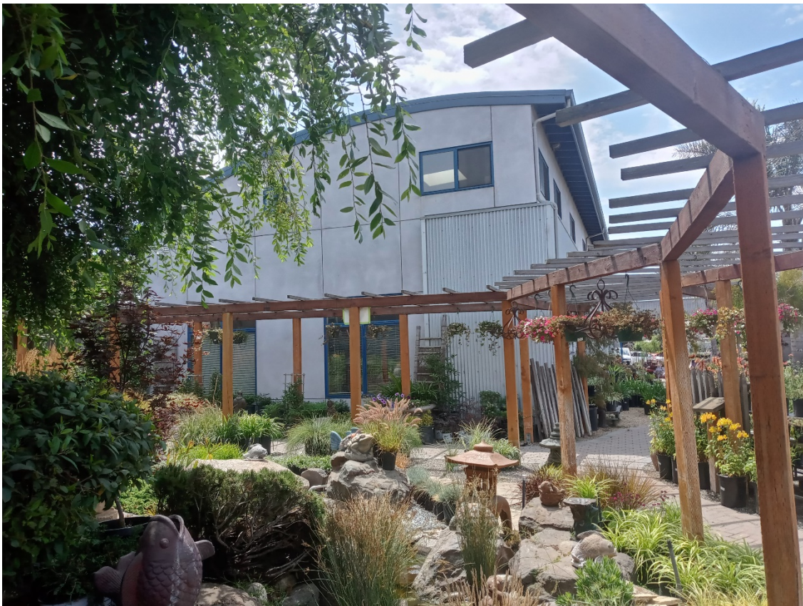
View of northern frontage, where stairwell to Caretaker Unit will be constructed (south).
