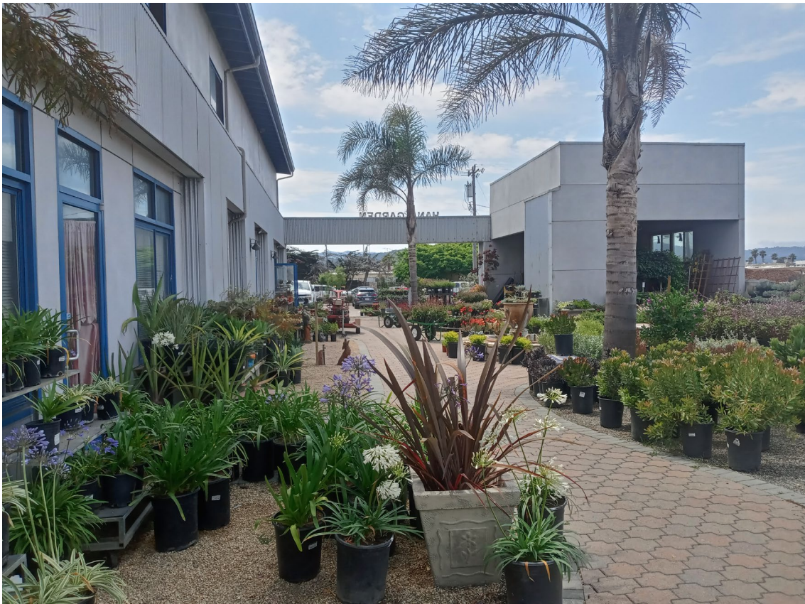
View of Building 1 (left) and Building 2 (right) looking south.
