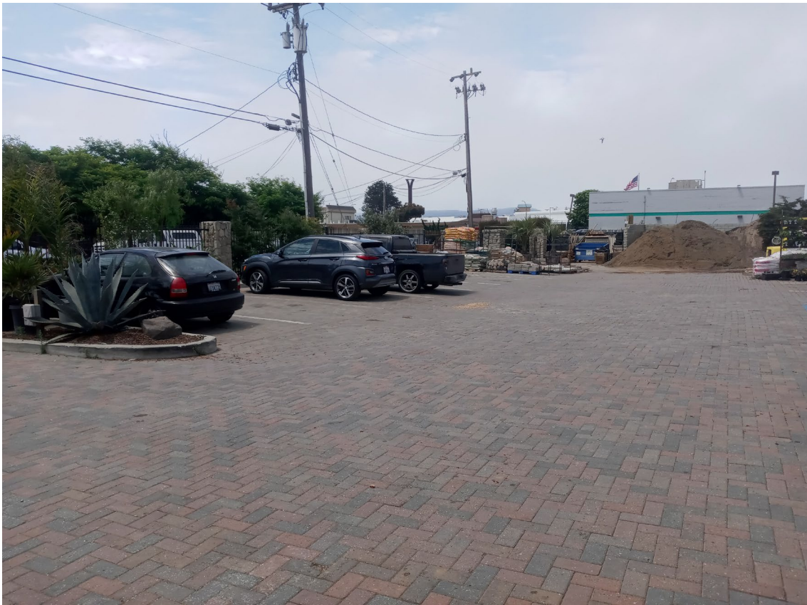
View of southern side of parking lot (west)
