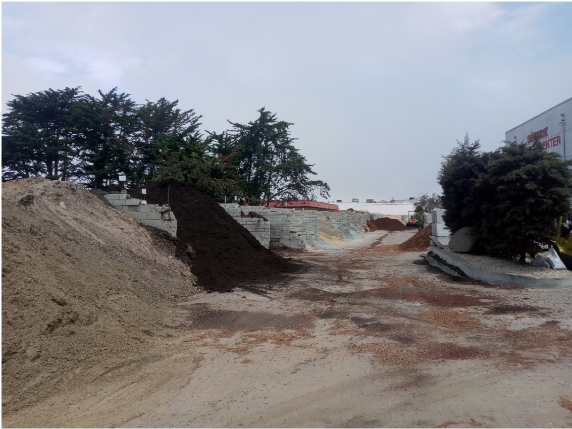
Materials storage on west side of property (north).
