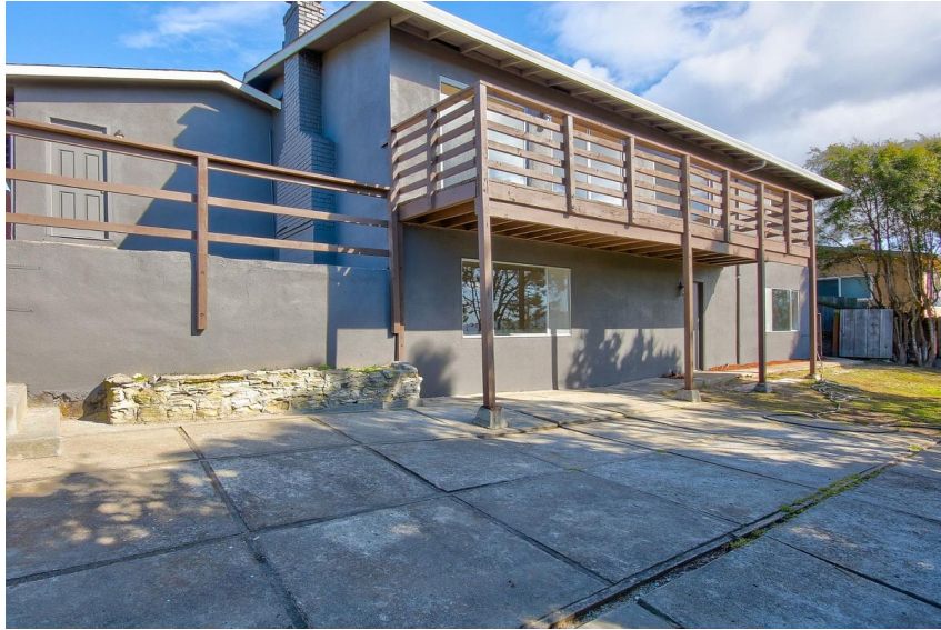
View of previous deck from north side of rear yard
