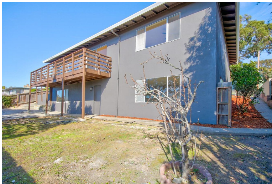
View of previous deck from south side rear yard
