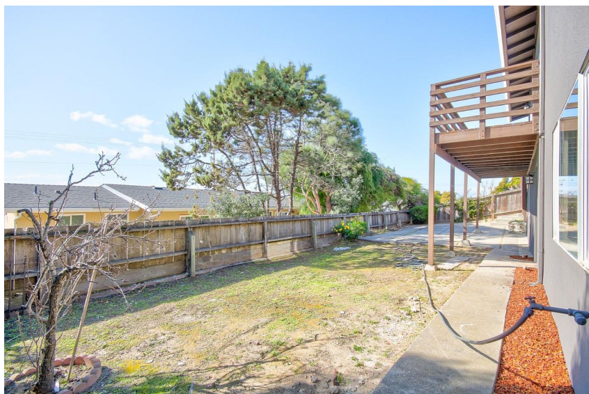
View of previous deck from south side of rear yard
