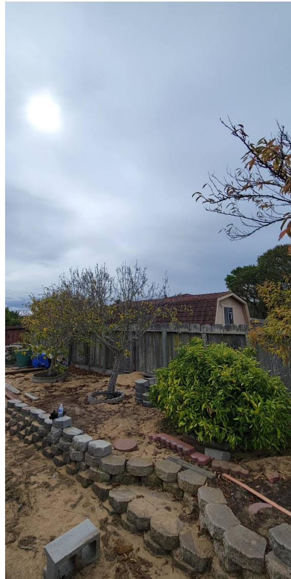
WEST ELEVATION/REAR YARD
