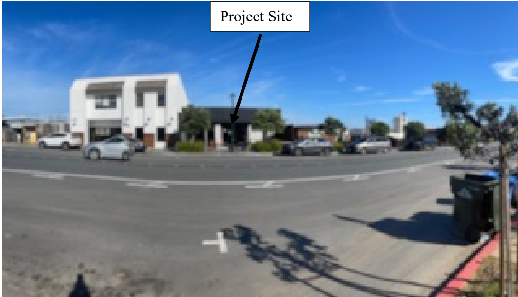
Front Façade facing Broadway Avenue
