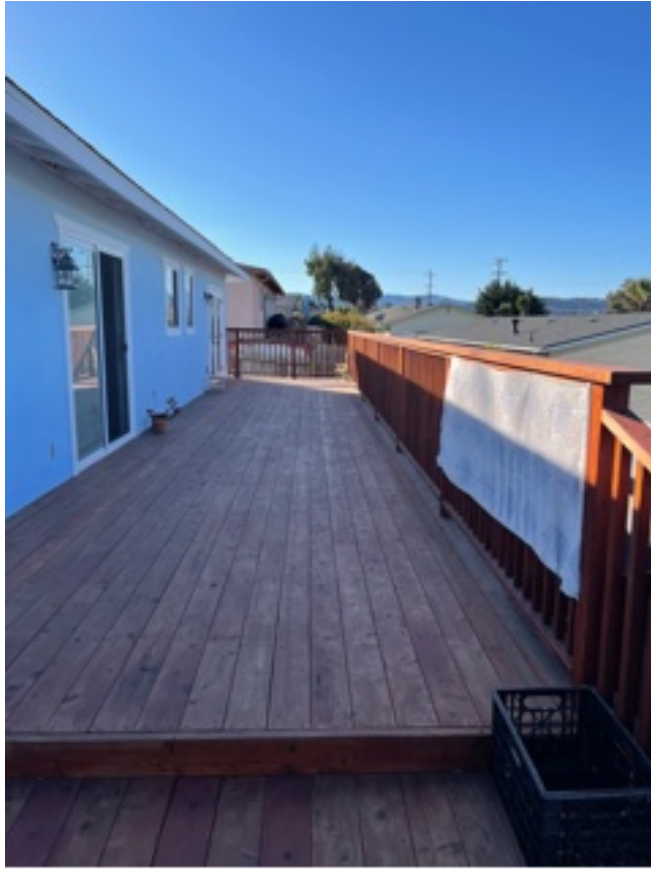
View of deck looking south
