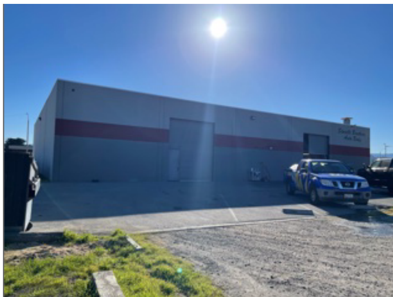
View of rear façade
