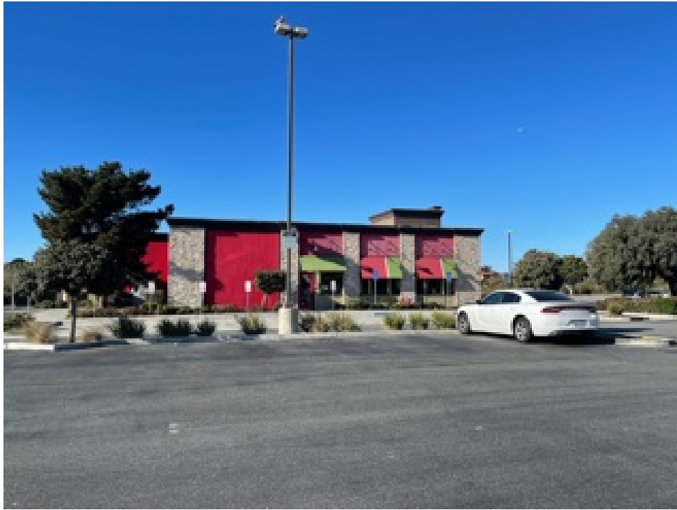
Façade facing Canyon Del Rey Blvd.
