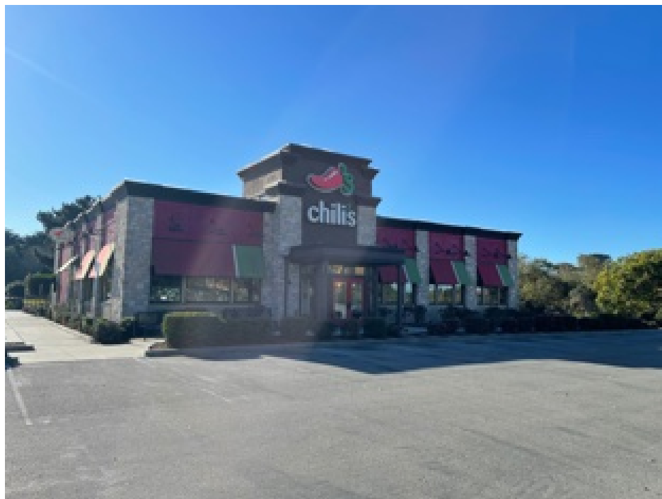
Front façade facing Embassy Suites Parking lot
