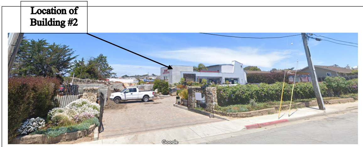
View from southwest corner looking north
