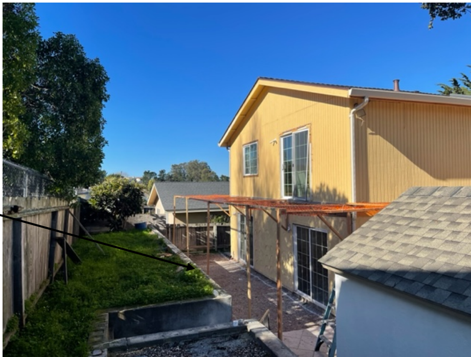
View of deck and stairway location looking west
