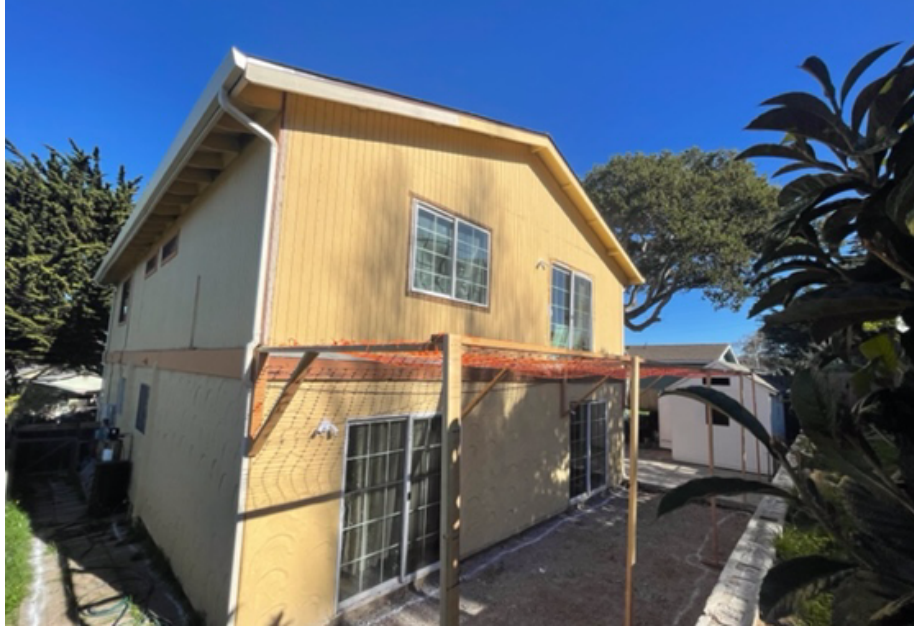
View of rear elevation looking east
