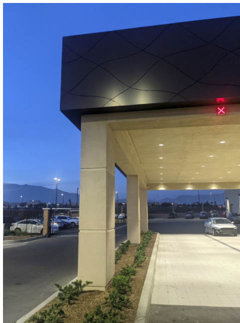
Image of Carport
