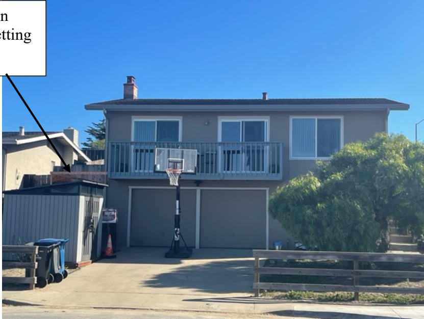
Western Elevation facing Yosemite Street
