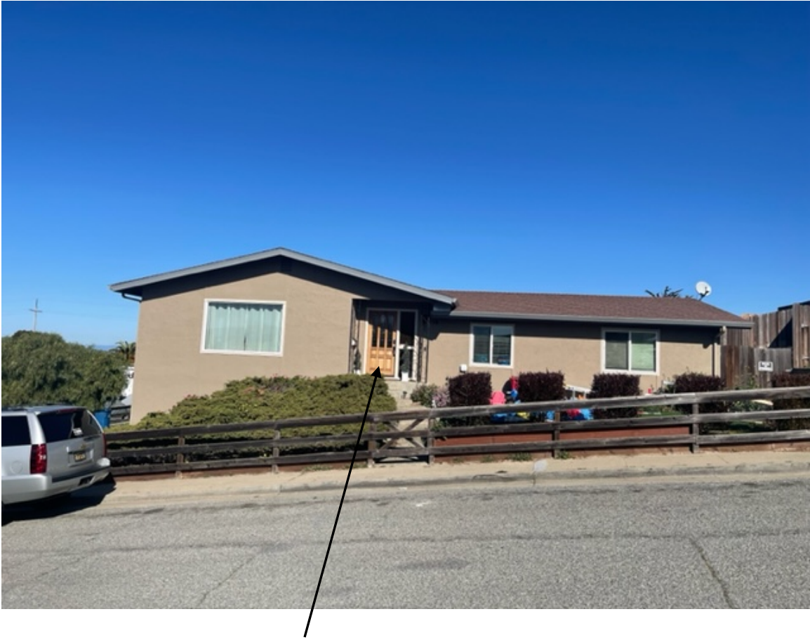
View of front entry access from Westminster Court
