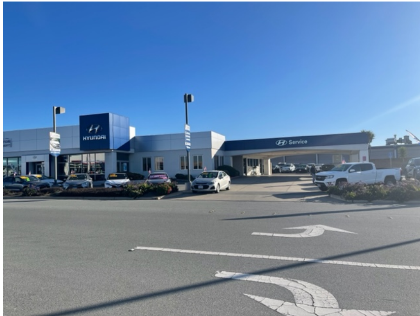
View of Showroom on west side
