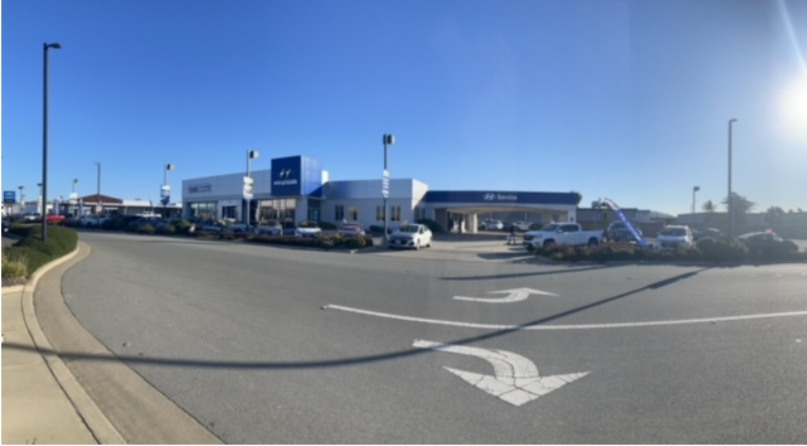
Panoramic View of Showroom
