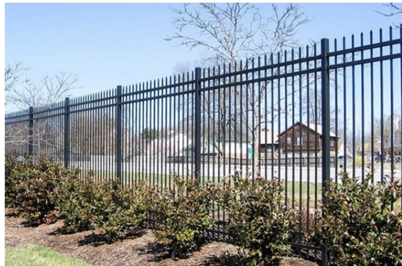
ORNAMENTAL 6' HI ALUMINUM PERIMETER FENCING
