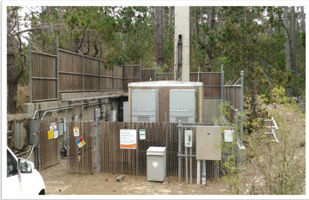
View looking north east
