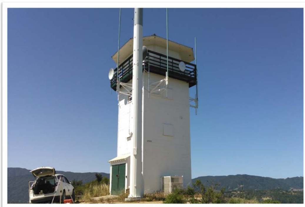
View looking south west at north face of building
