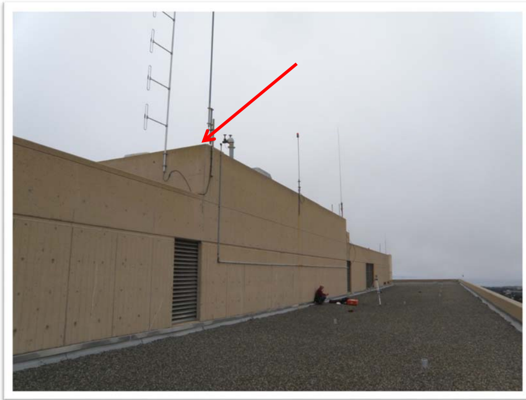
View looking south west at penthouse standing on main roof level *Arrow points to proposed location for antenna to E911
