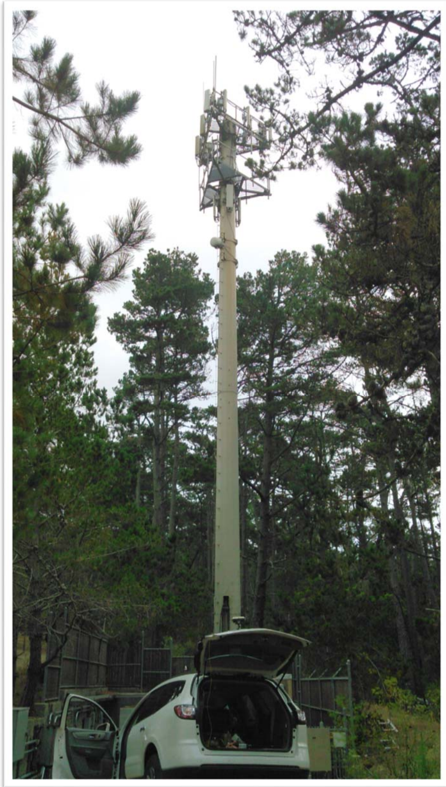
View looking north east
