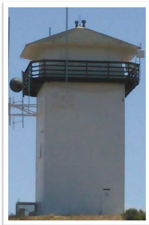
View looking east at west face of building
