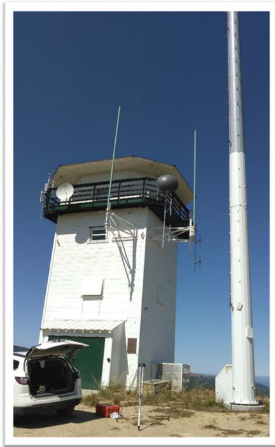
View looking west at east face of building
