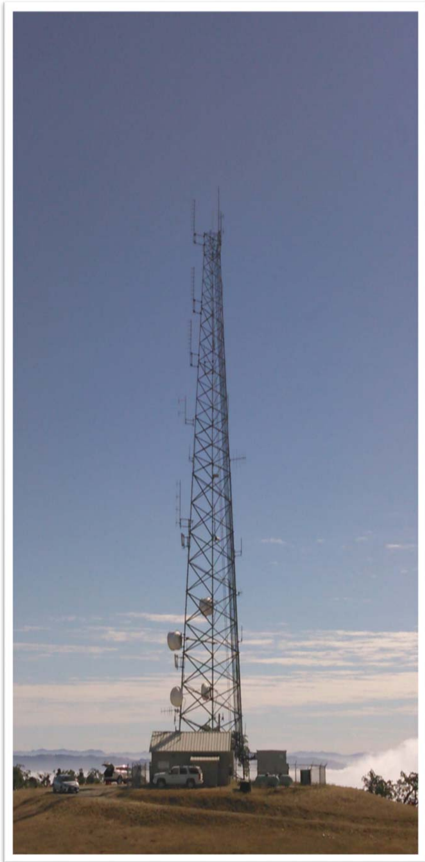
View looking north easterly of tower
