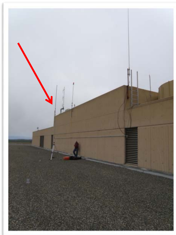
View looking south east at penthouse standing on main roof level
