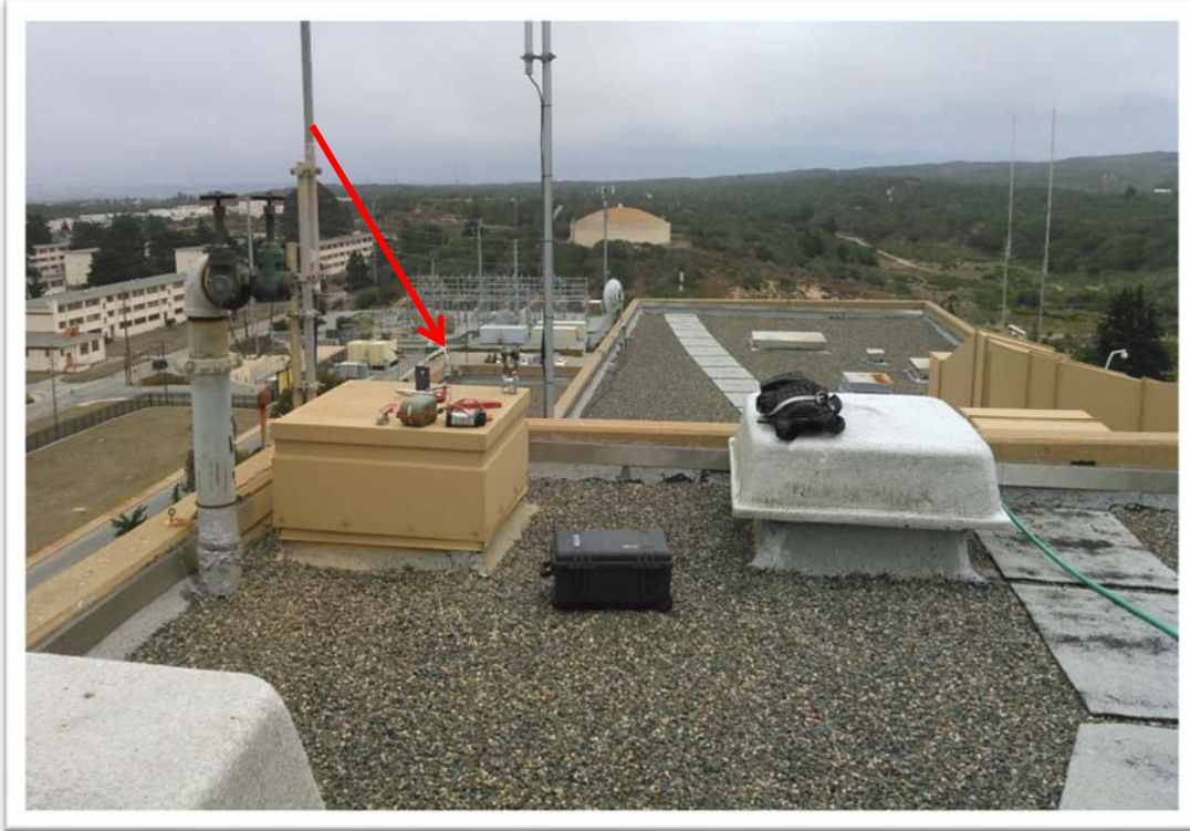
View looking westerly standing on upper penthouse *Red arrows point to proposed antenna location
