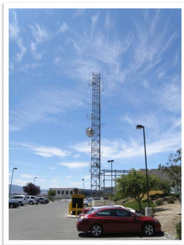
View looking southerly
