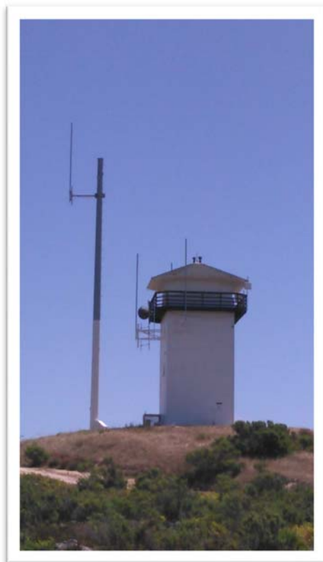
View looking east at west face of building
