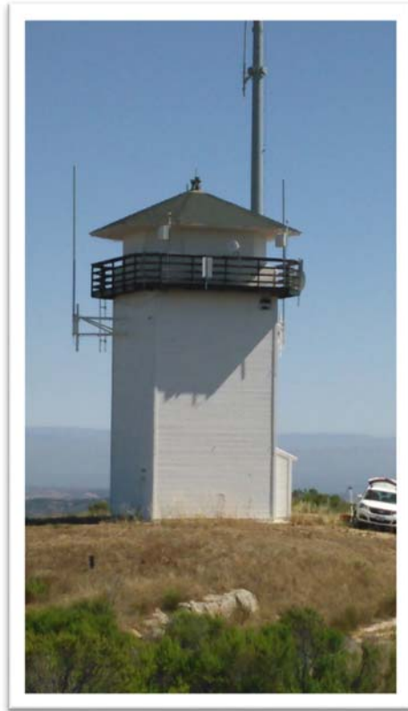
View looking north at south face of building
