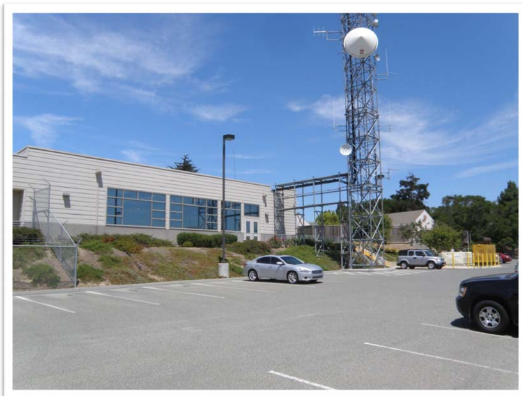
View looking north westerly
