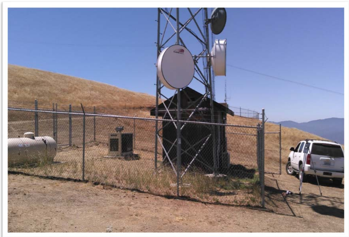
View looking south easterly
