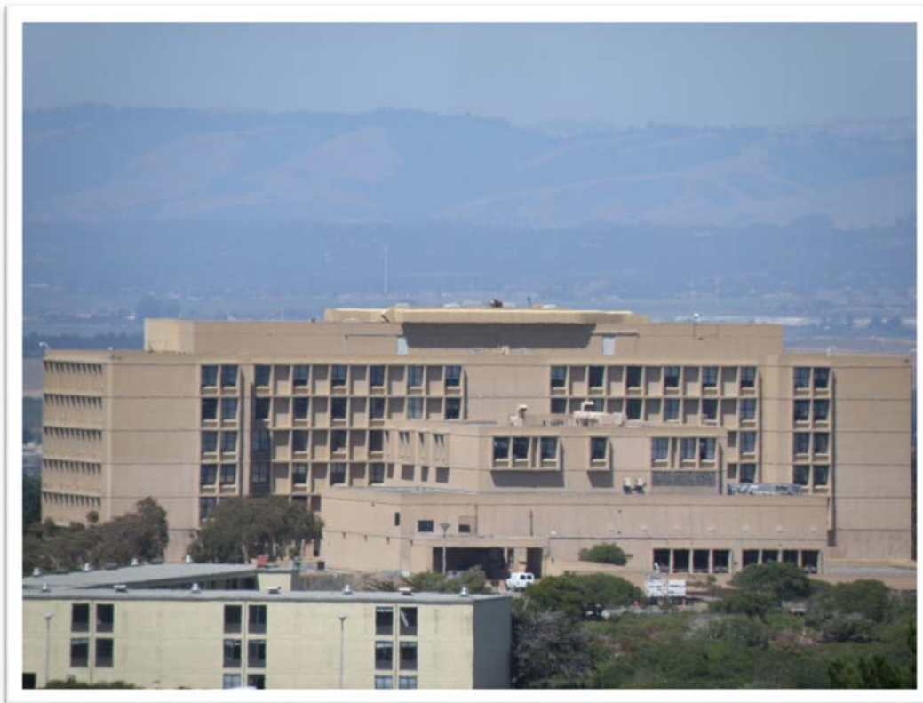
View looking northerly at south face of DOD building
