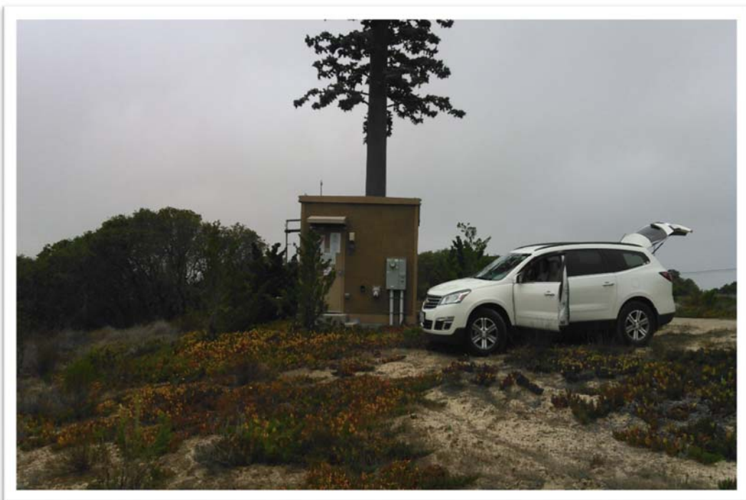
View looking north westerly
