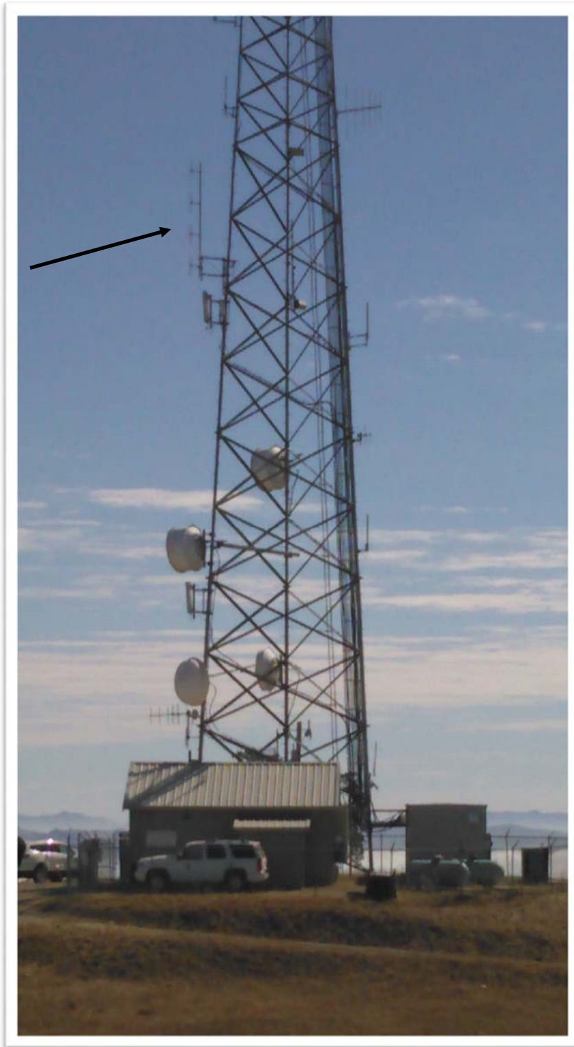
View looking north easterly lower tower *Arrow points to dipole needing relocation
