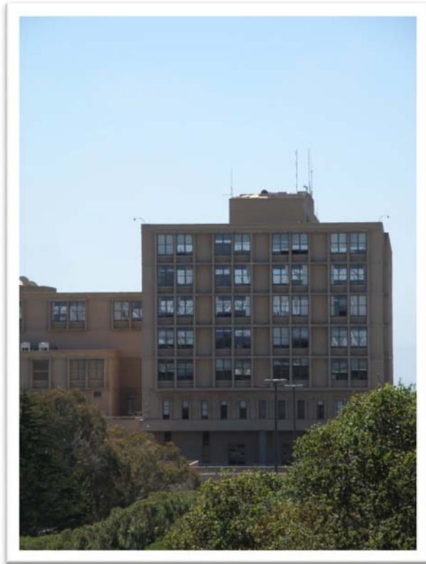
View looking westerly at east end of DOD building
