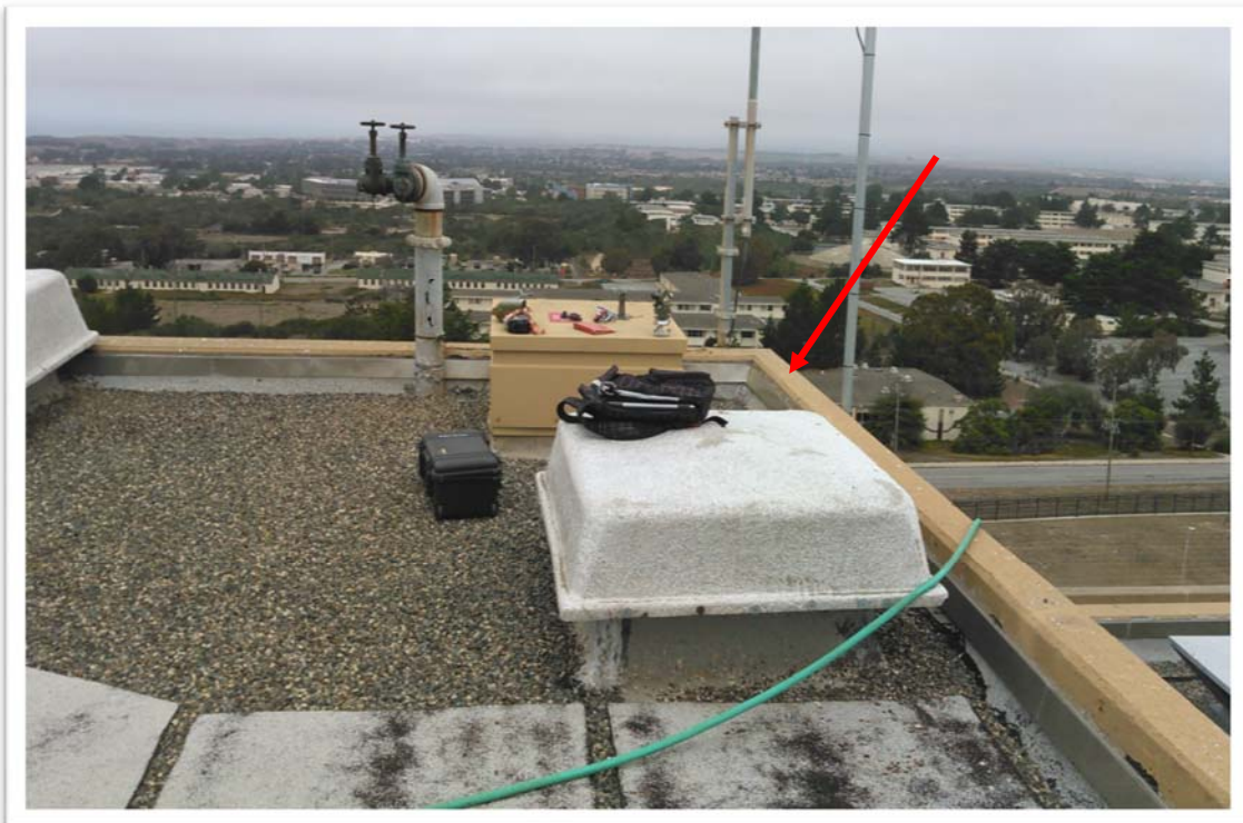
View looking northerly on upper penthouse level
