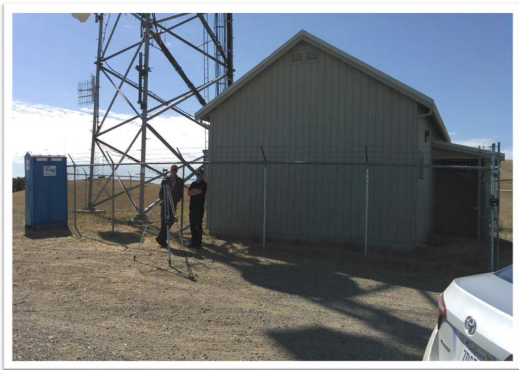
View looking southerly
