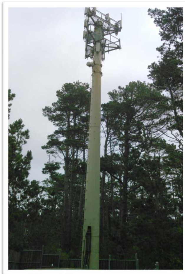
View looking north east
