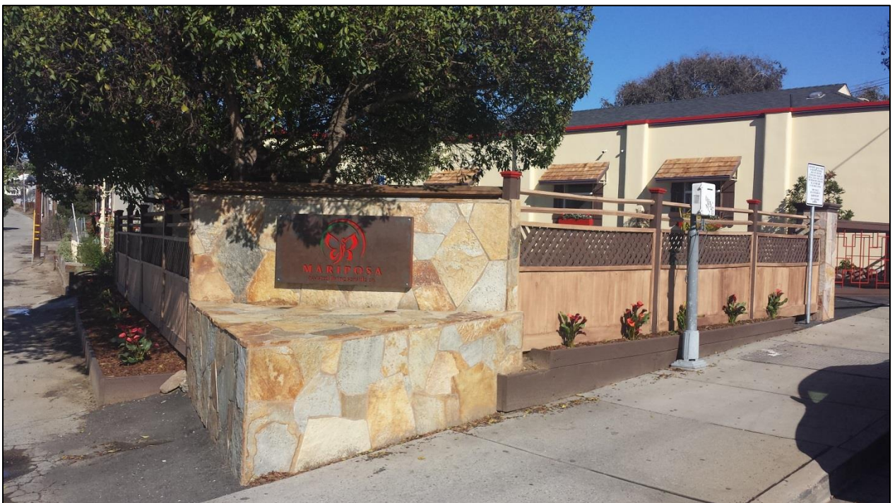
View of Project Site After Installation of Sign
