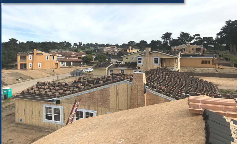
New homes under construction in Seaside 2022
