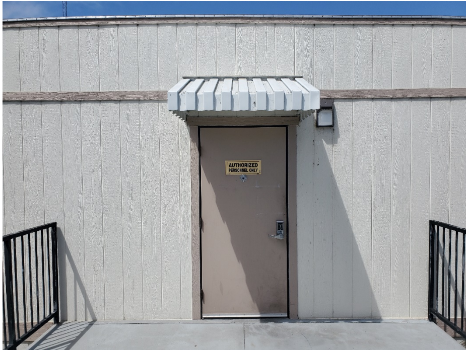
Photo exhibit for existing exterior finishes
