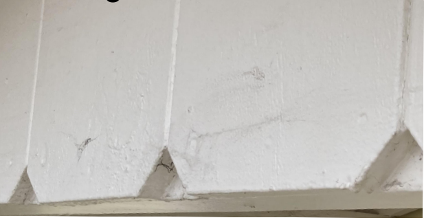
Upper siding: vertical white wood siding
