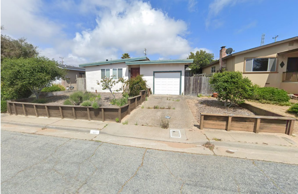
Driveway at 1836 Juarez Street
