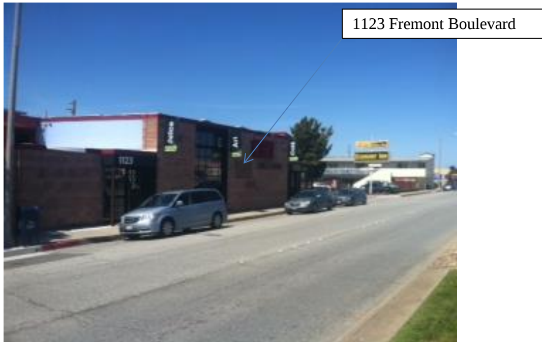
View of front façade of project site from Fremont Boulevard
