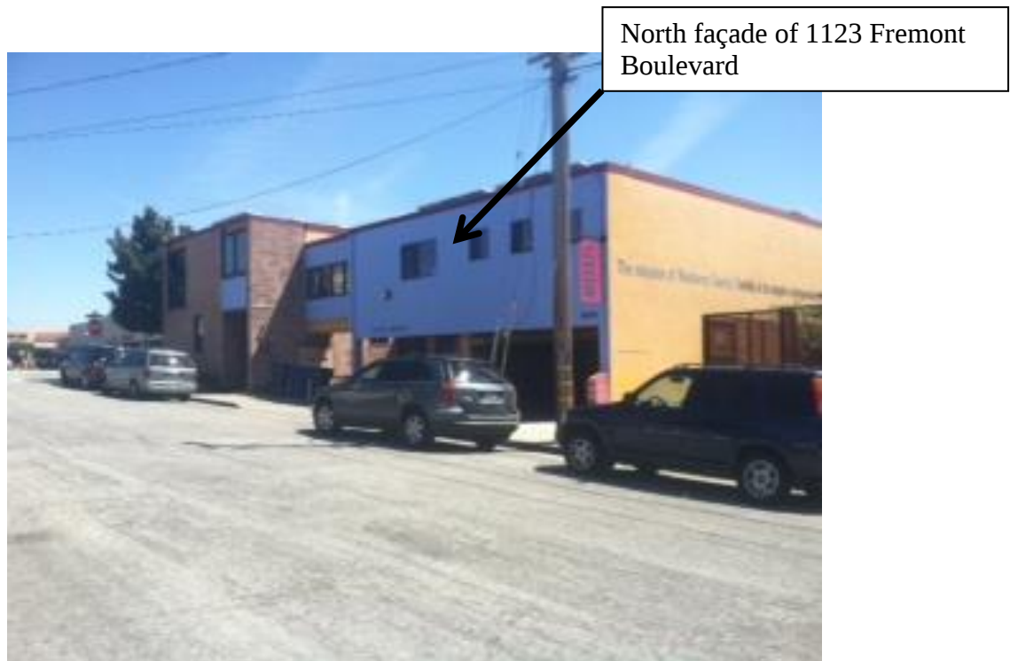
View of the north façade of 1123 Fremont Boulevard as seen from Williams Avenue
