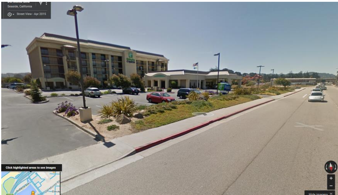
View of front elevation looking south from Del Monte Boulevard
