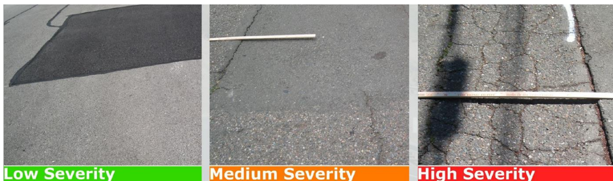
Image 5: Patching and Utility Cut Patching
