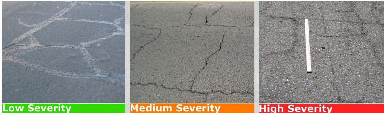
Image 2: Block Cracking
