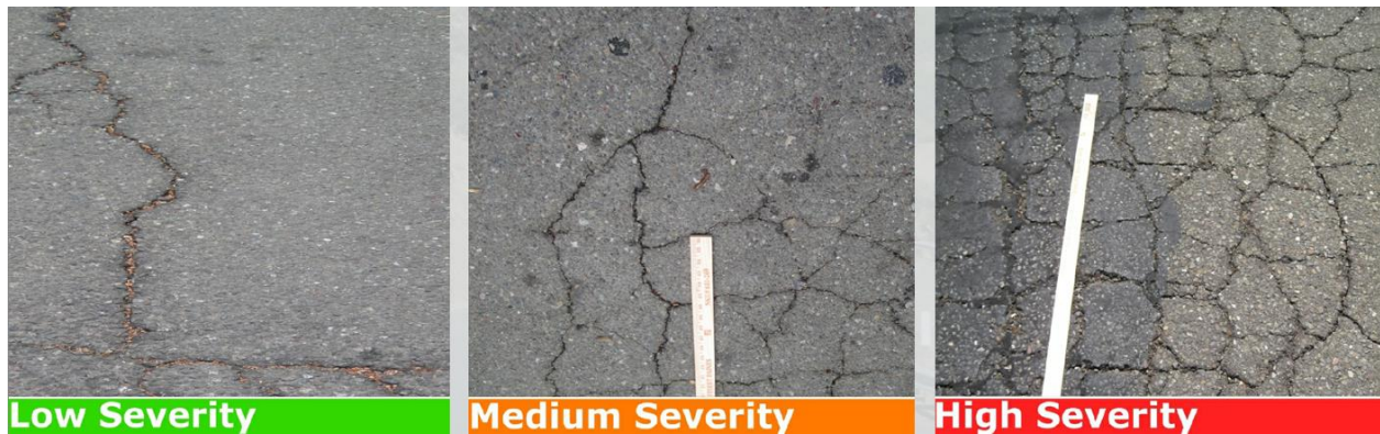
Image 1: Alligator Cracking
