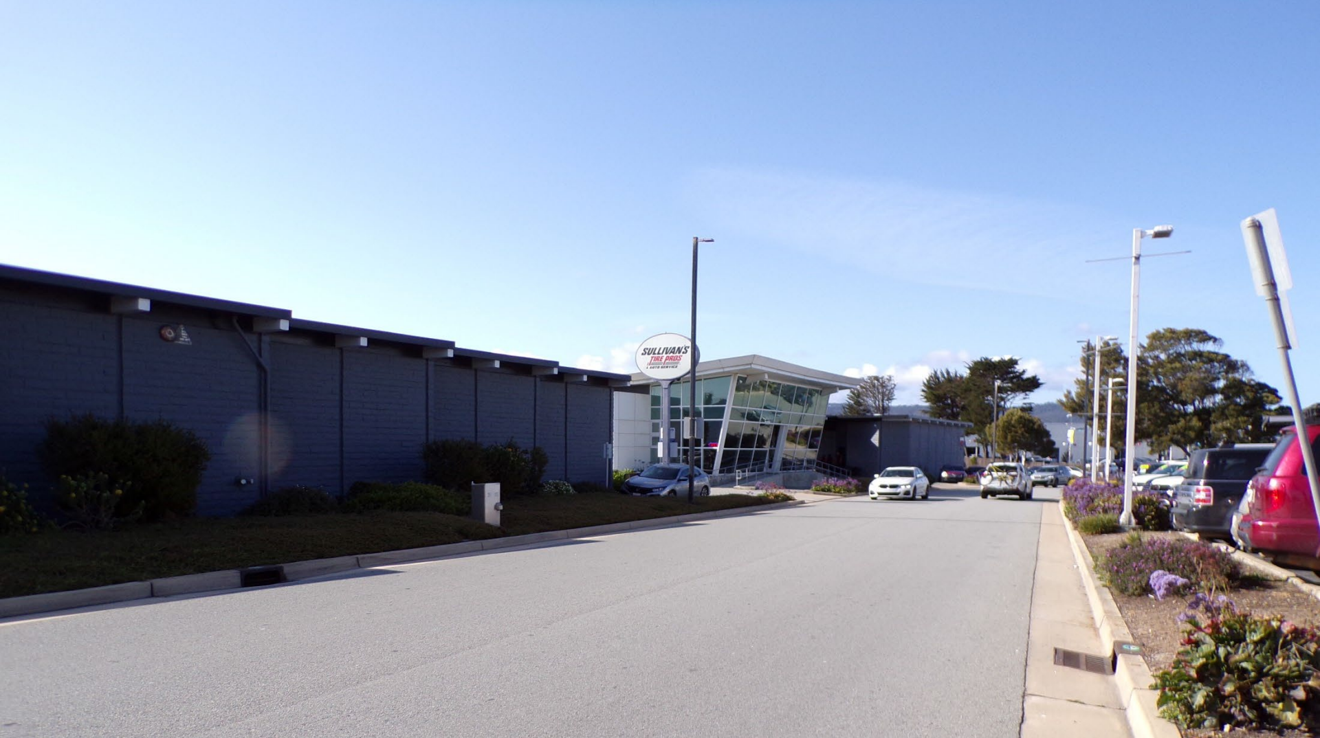
Image 3: The image shows Sullivan's Tire from the northern approach on The Mall. Three buildings are shown, on the left and closest to the viewer is the short two-toned grey building. The next closest structure is the tall pylon sign. From this angle the sign is clearly taller than the short building and a similar height to the central building with glazing and white cornices, which is slightly farther away. In the back right of the image, the final two-tone grey building is just visible.
