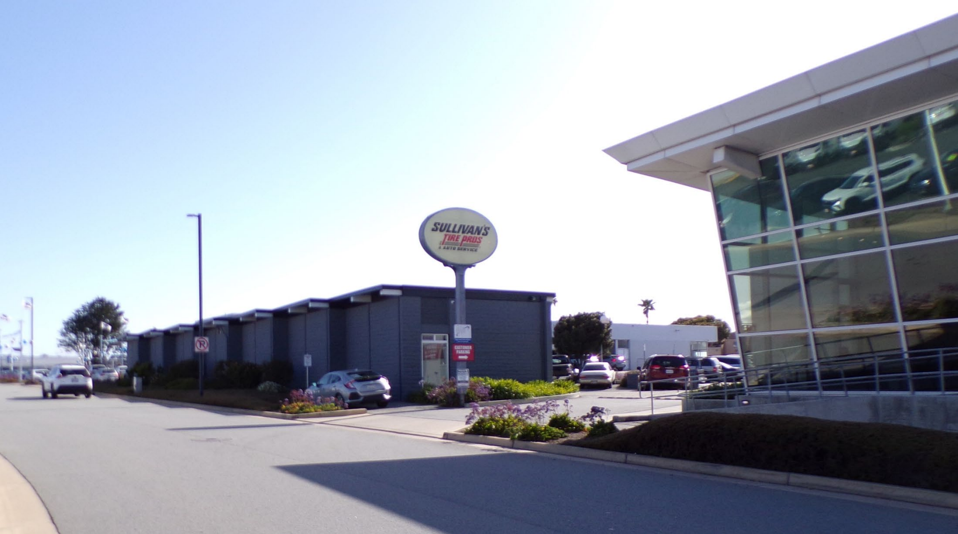
Image 2: The image shows Sullivan's Tire from The Mall. The existing pylon sign is shown in the center of the photograph, clearly taller than the short building painted in two tones of grey. Some cars are parked nearby but are not close enough to the sign for a direct comparison. The right of the photograph shows part of the tall building that is finished in glazing with a white cornice. The building is closer than the pylon sign, making relative heights difficult to judge.
