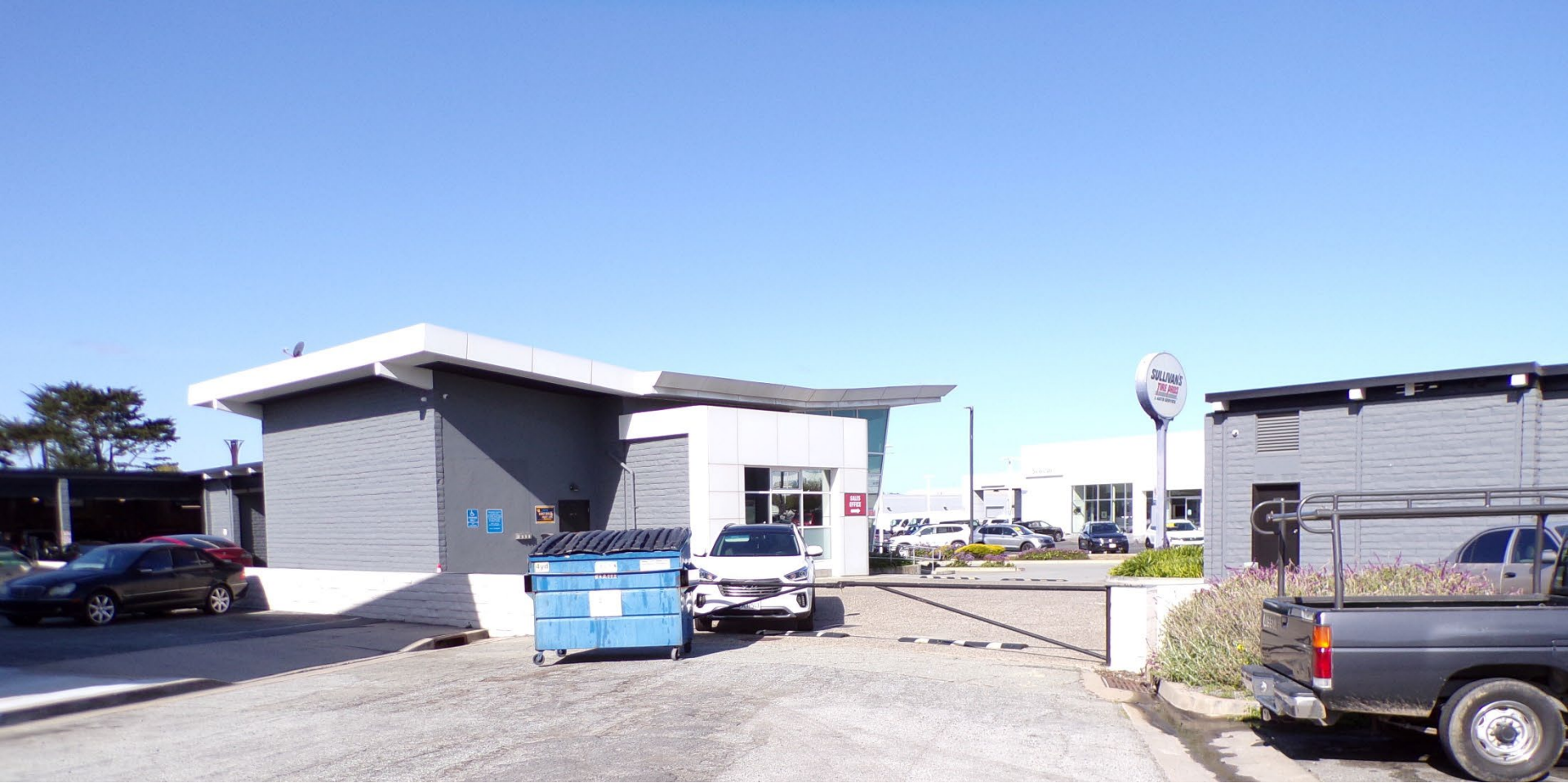
Image 4: The image shows the rear of the central building from the eastern end of Columbus Ave. Some of the glazing can be seen but it's mostly hidden by the angle of the photograph. The building is painted great with white panels. A dumpster blocks part of the view and a gate bars access to the parking lot. In the background, the existing pylon sign can be seen. From this angle it is approximately the same height or taller than the central building. Part of the northern two-tone grey building can be seen in the extreme right of the photograph. This is the location where sign #2 is proposed to be installed.
