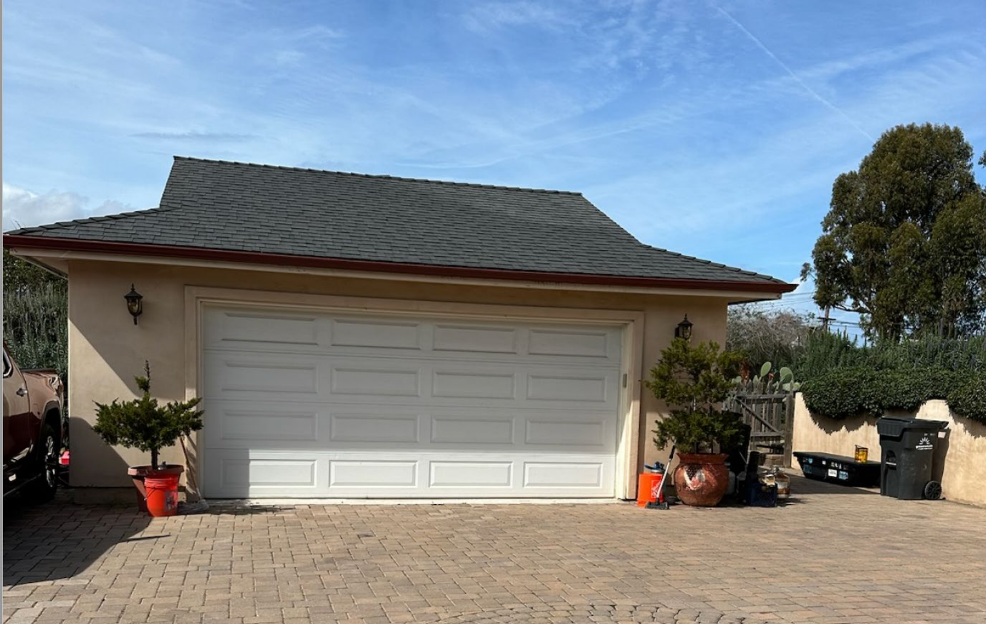
Image 2. View of the existing garage
