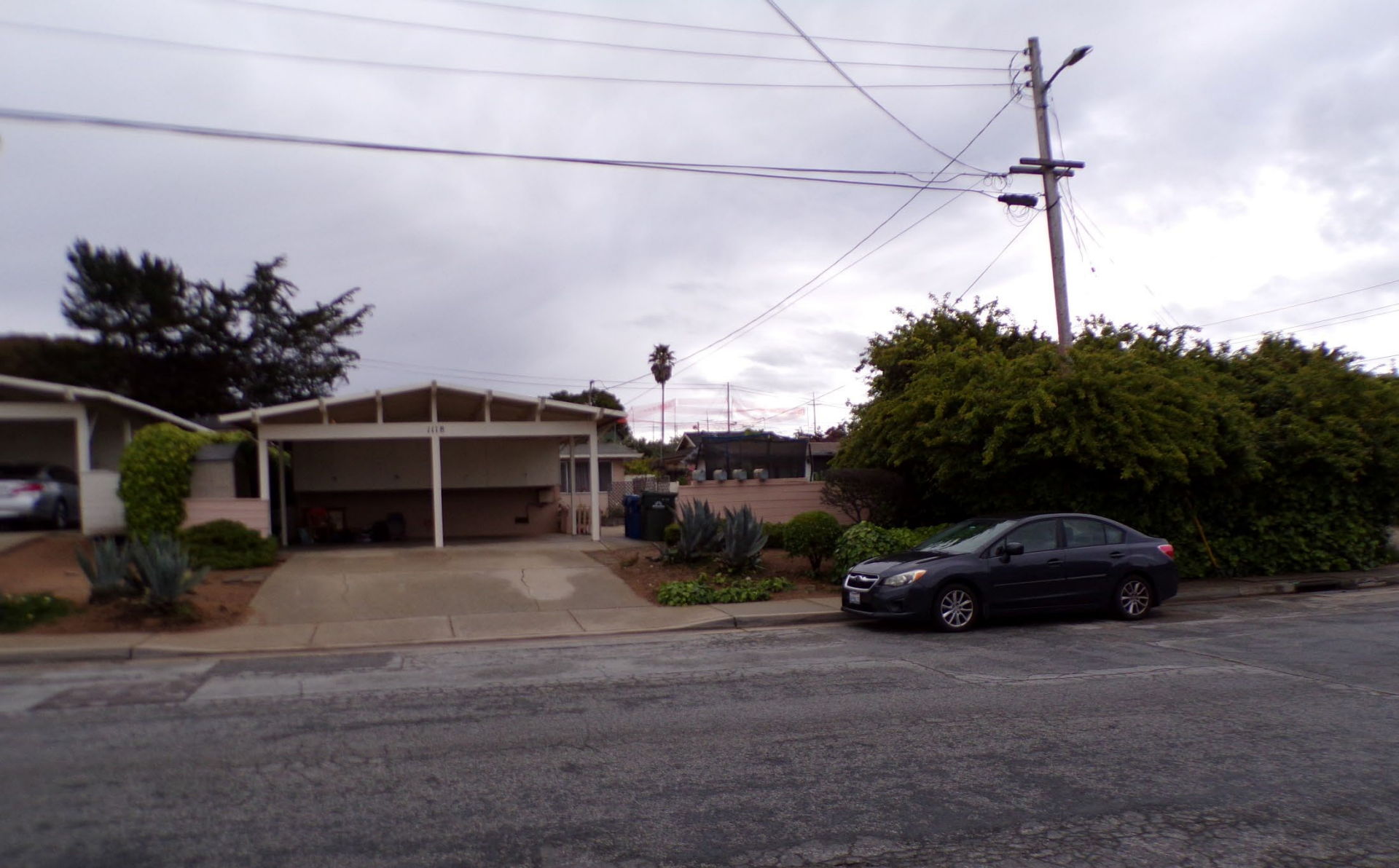
Image 12. View of flagging from Waring Street.
