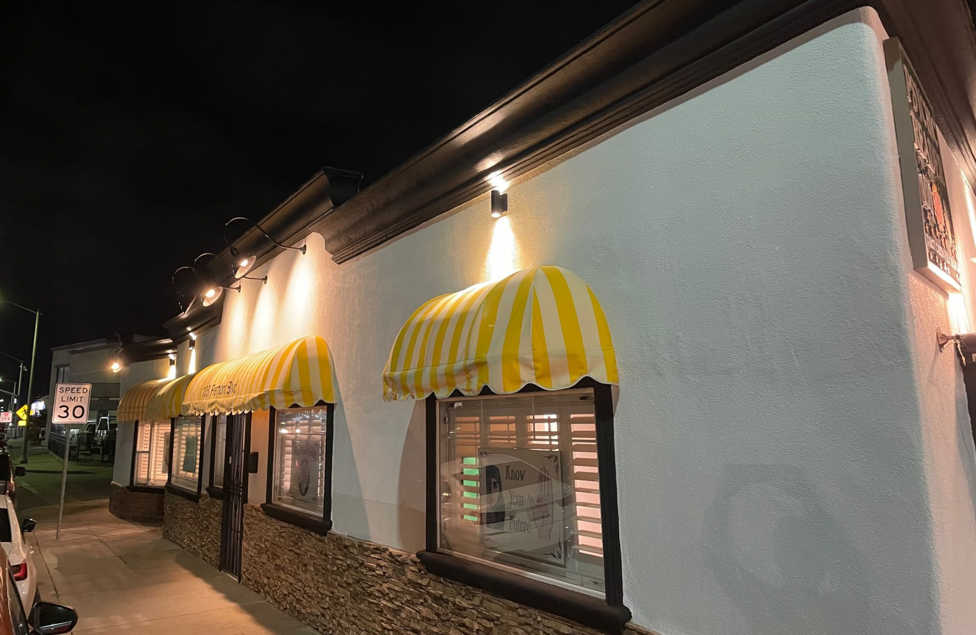
Photo 2. Facade facing Fremont Boulevard from the north.
