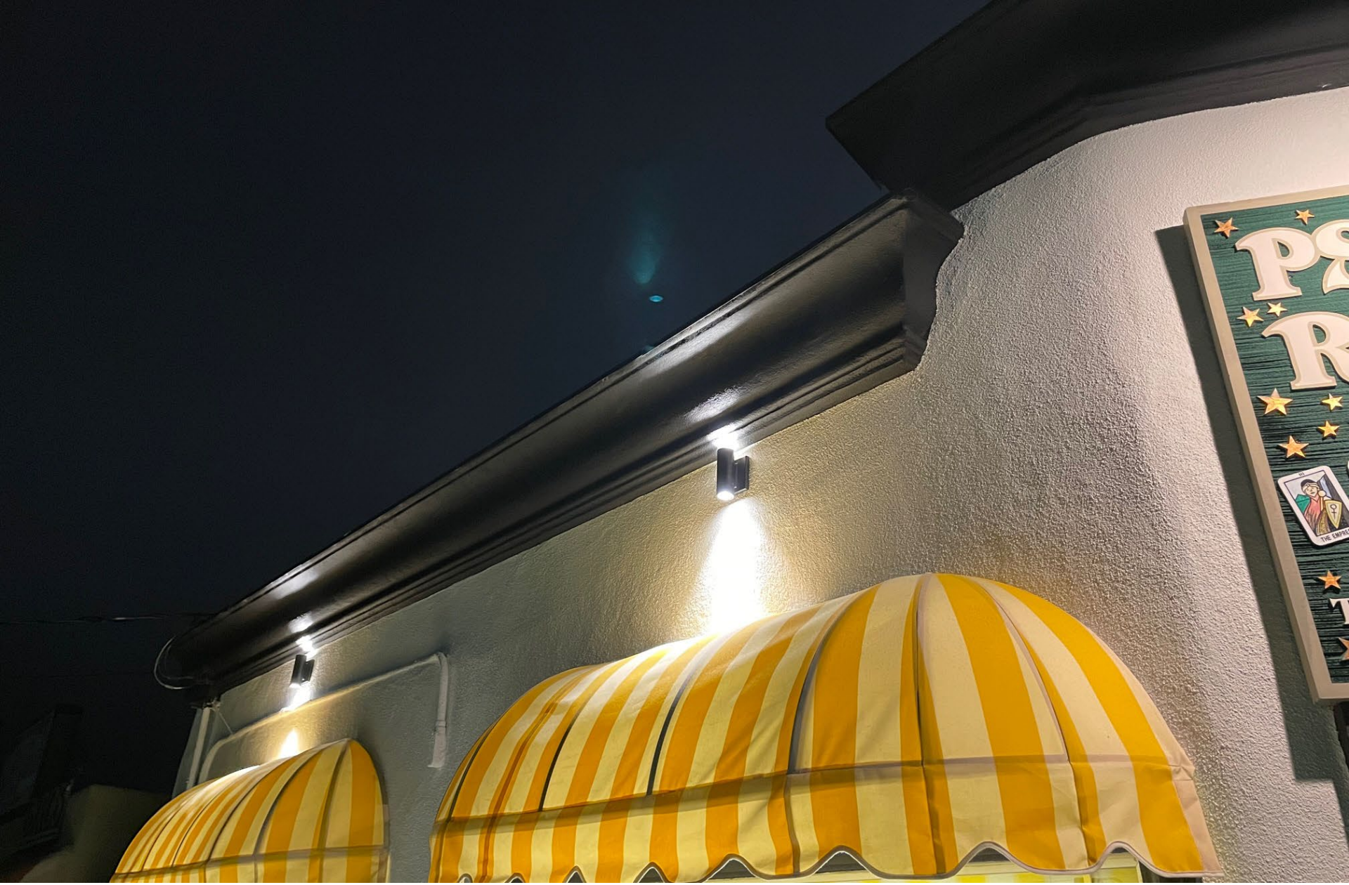
Photo 3. Close-up of uplighting.
