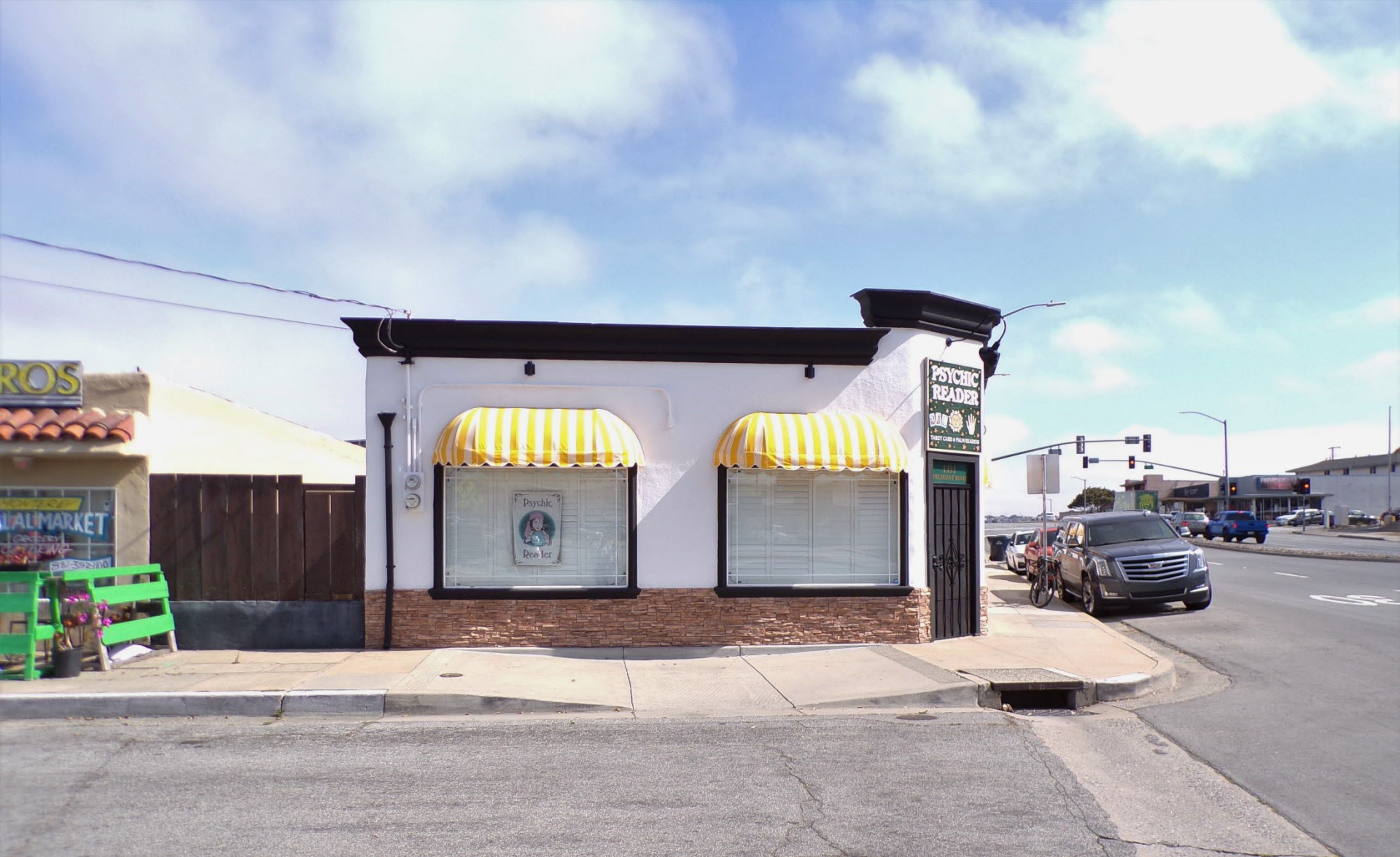
Photo 2. South façade facing Hamilton Avenue.
