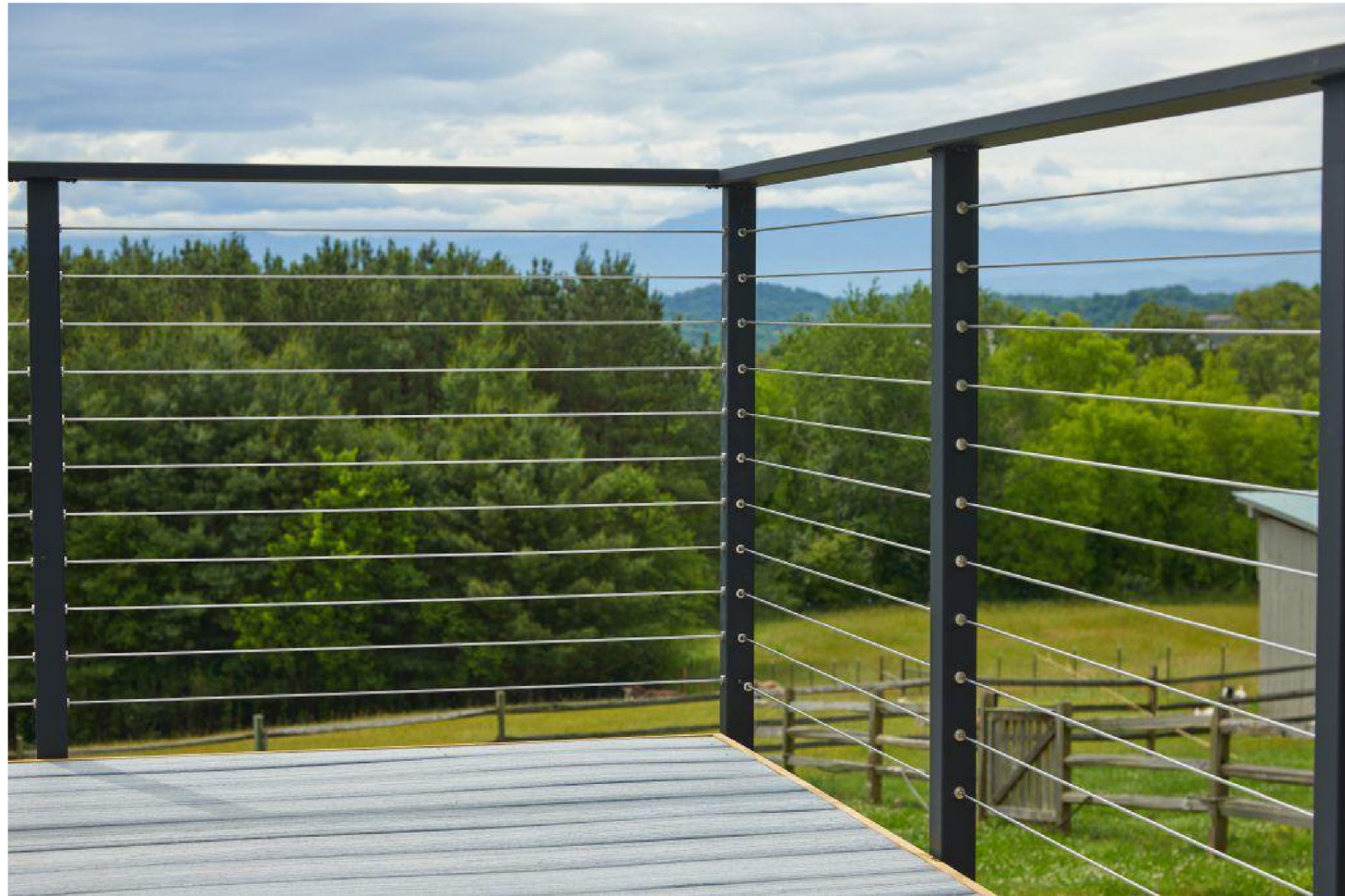
NEW METAL CABLE RAILING SYSTEM @ PROPOSED DECK
