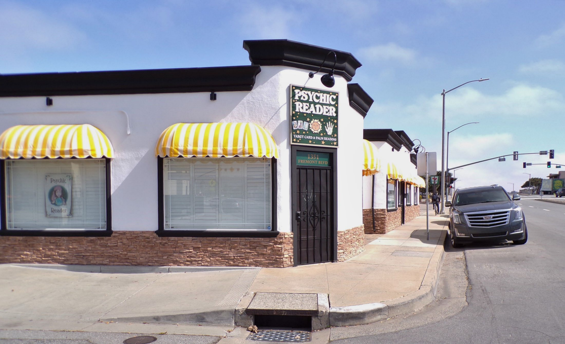
Photo 1. Overview of façade.
