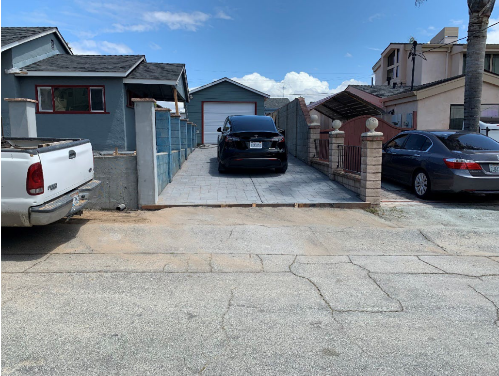
Existing driveway on Kenneth.
