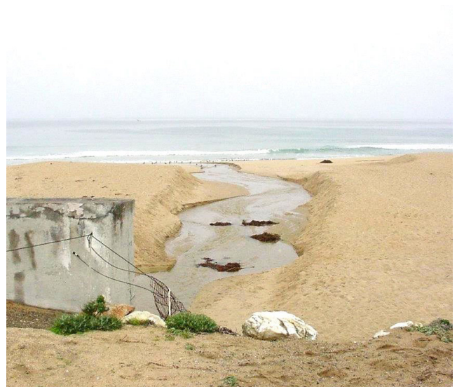
Stormwater Outfall in Seaside.
