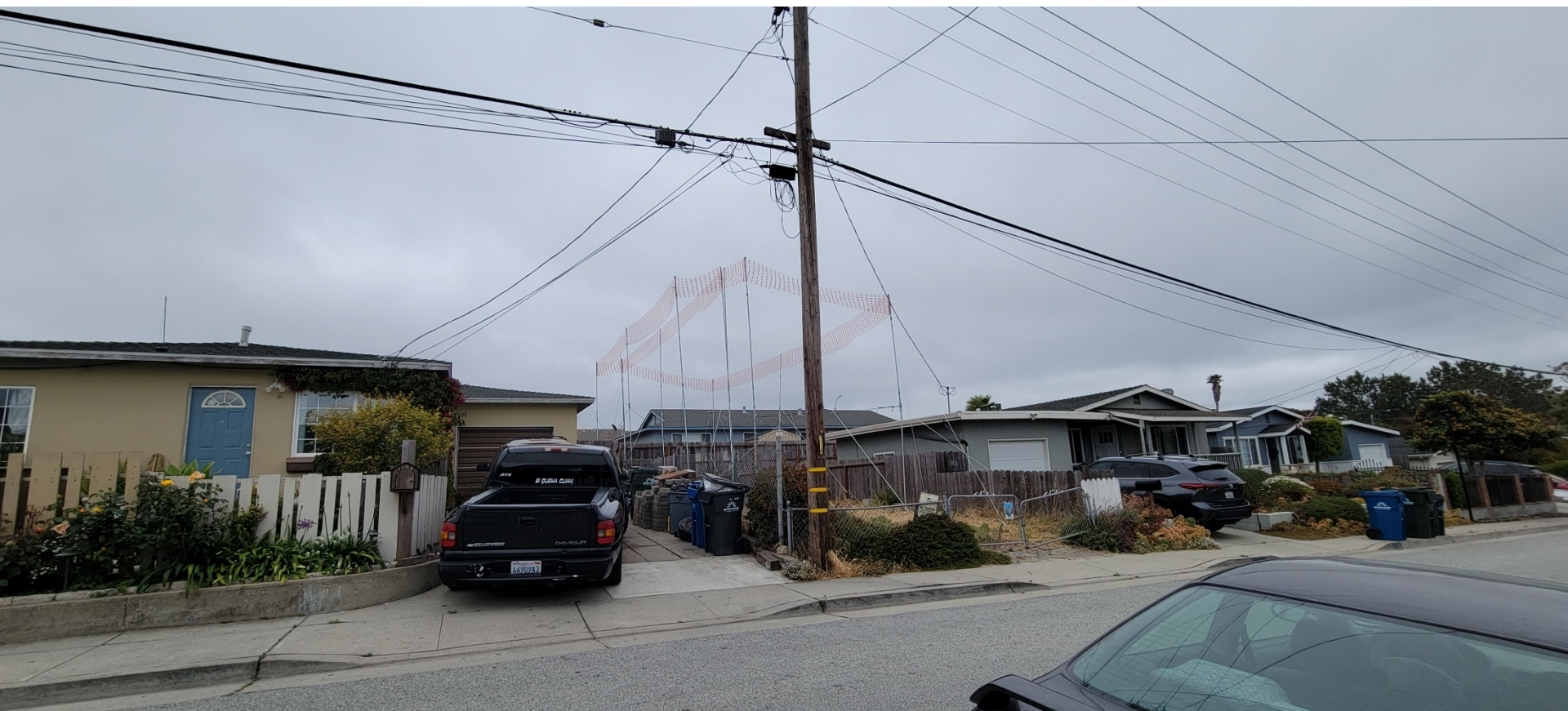
Image 2. View from Laguna Avenue looking east directly at the flagging of 1784 Laguna Street. The flagging is taller than nearby buildings.
