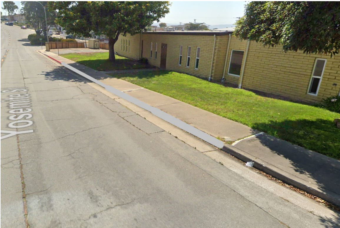
Yosemite St. – Paint 97 feet of curb gray. Leave 20 feet of curb red, nearest parking lot exit.
