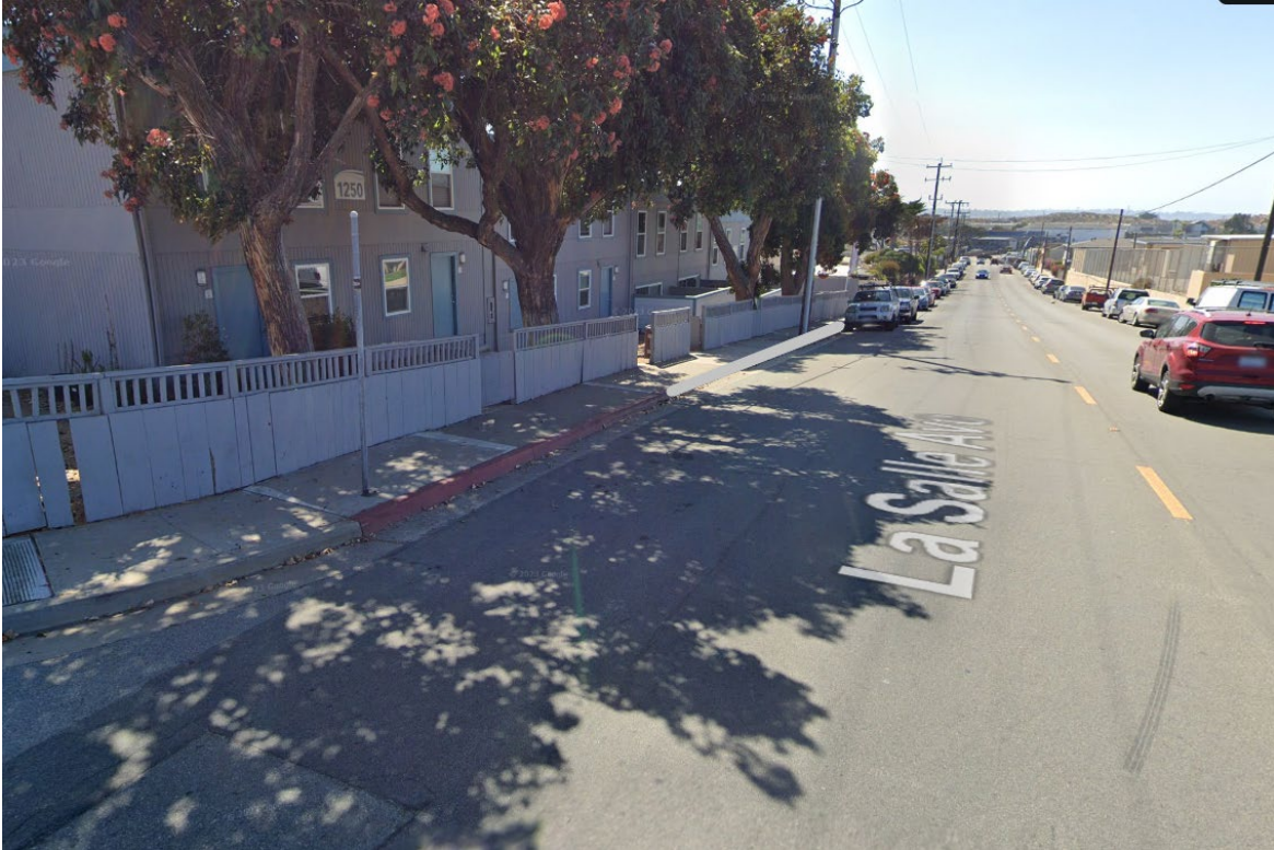
La Salle Ave. – Paint 70 feet of curb gray. Leave 20 feet of curb red, nearest intersection.
