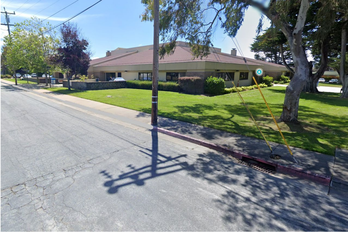
Wheeler St. - Paint 120 feet of curb gray. Leave 20 feet of curb red, nearest intersection.
