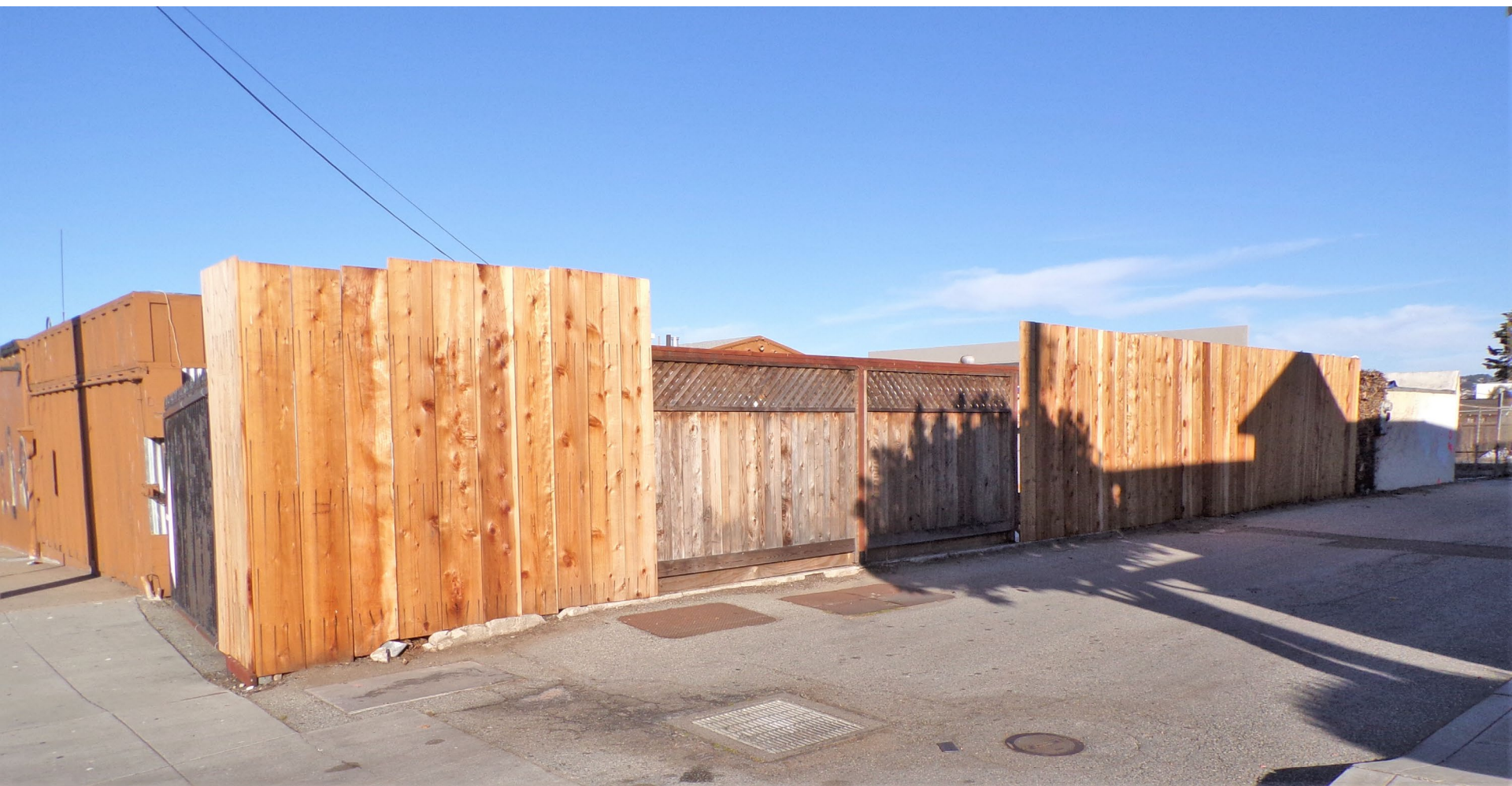
Picture 3: View of 500 and 510 Broadway Ave. from the alley at the rear of the property.
