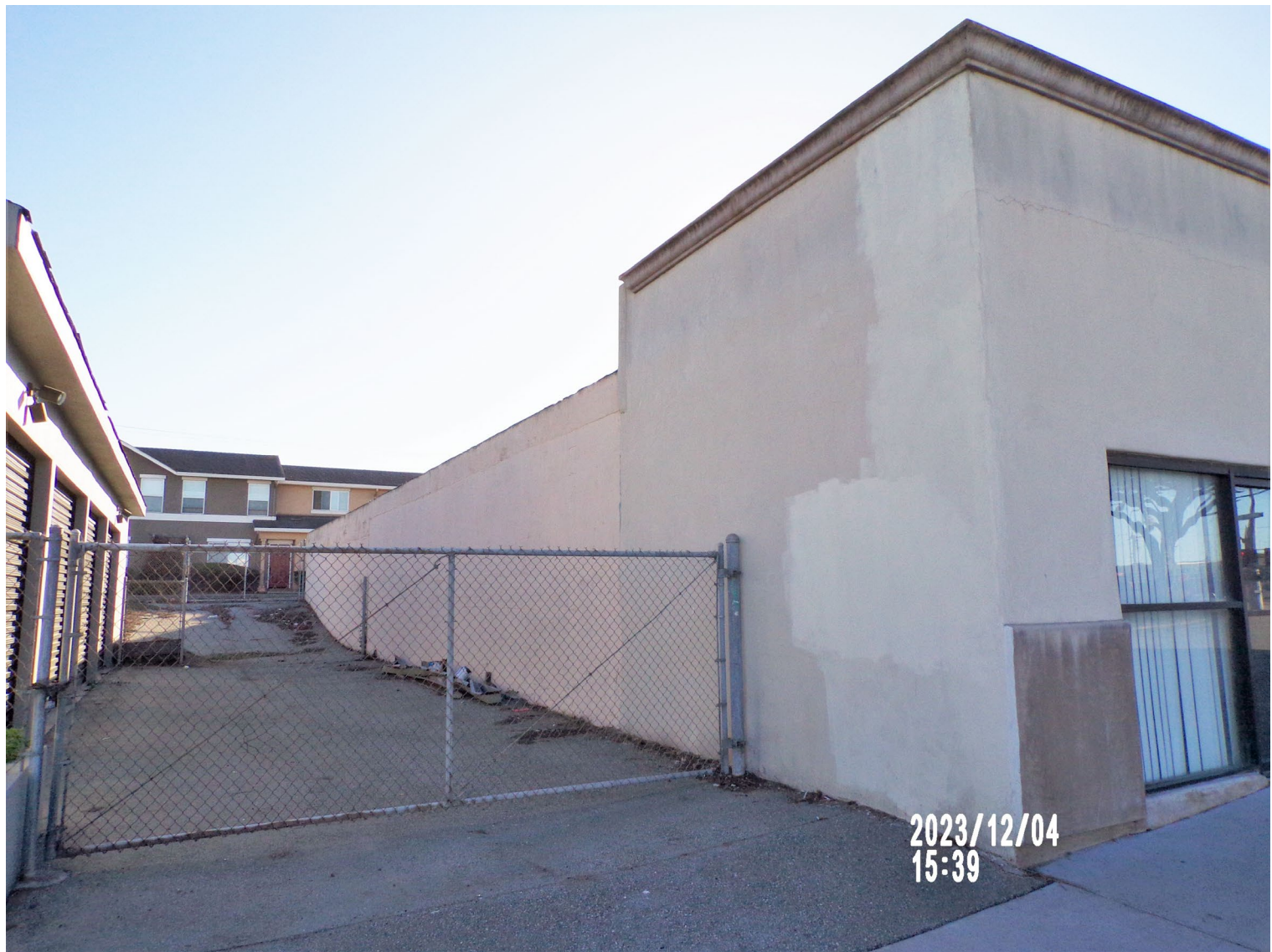
Picture 4: View of 510 Broadway Ave. showing the east side of the building.
