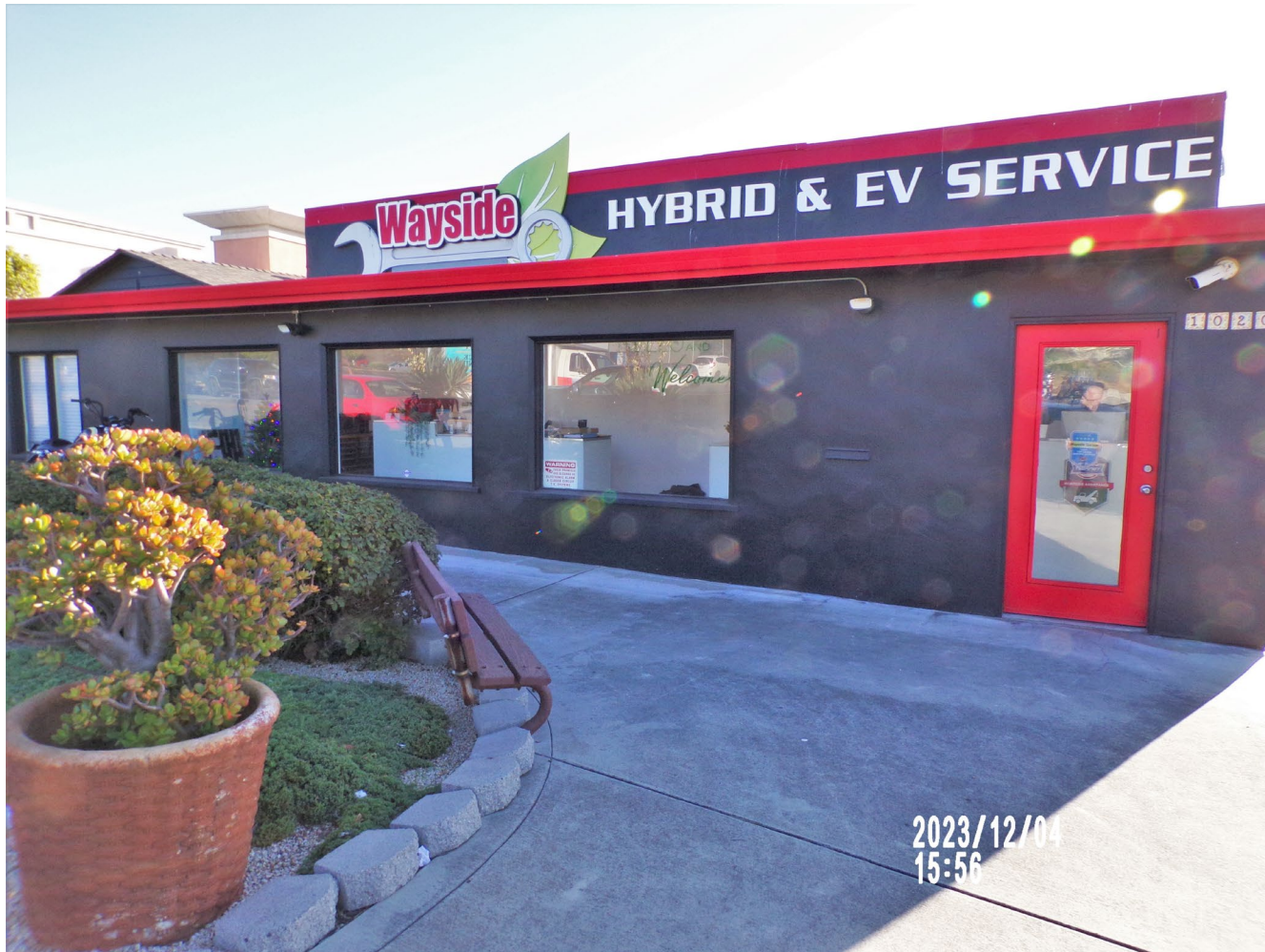
Picture 5: View of Wayside Garage from the sidewalk along Ord Grove Ave.
