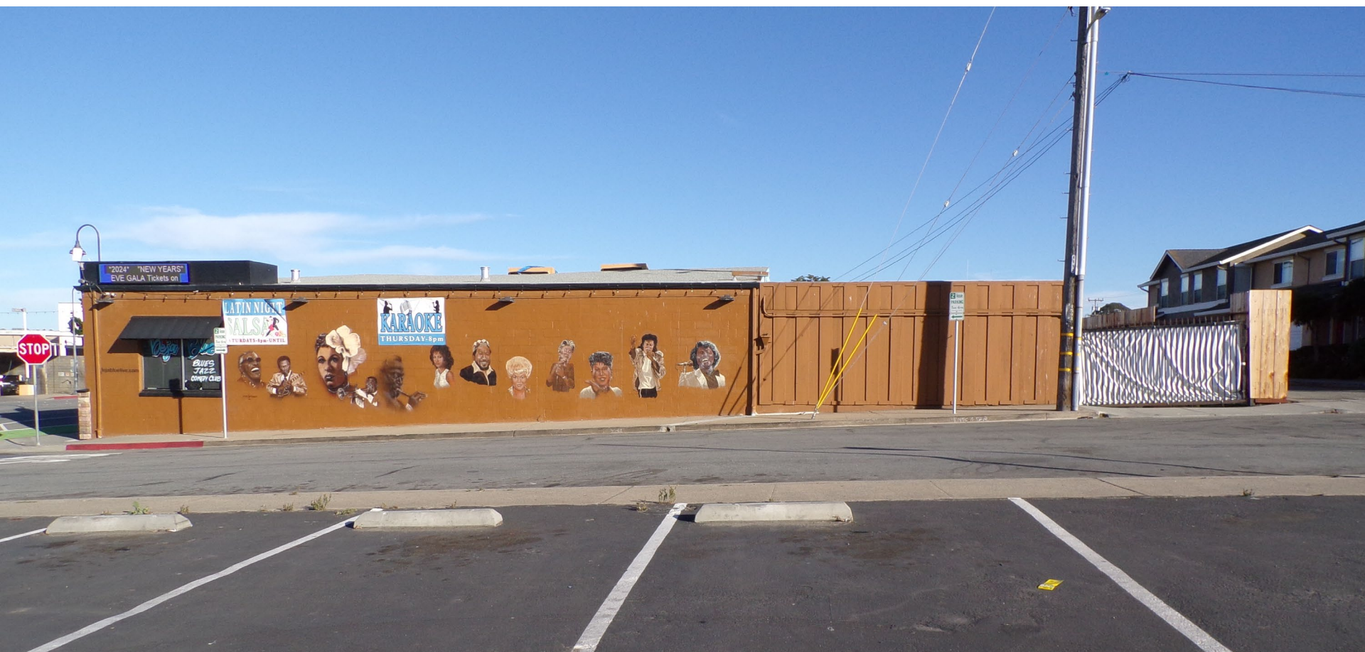
Picture 2: View of the Contra Costa St. frontage (west side).
