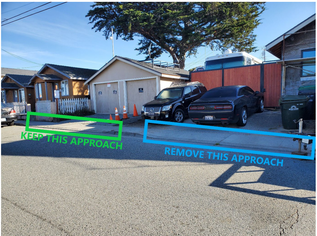
Area of existing driveway approaches, on Hilton Street.
