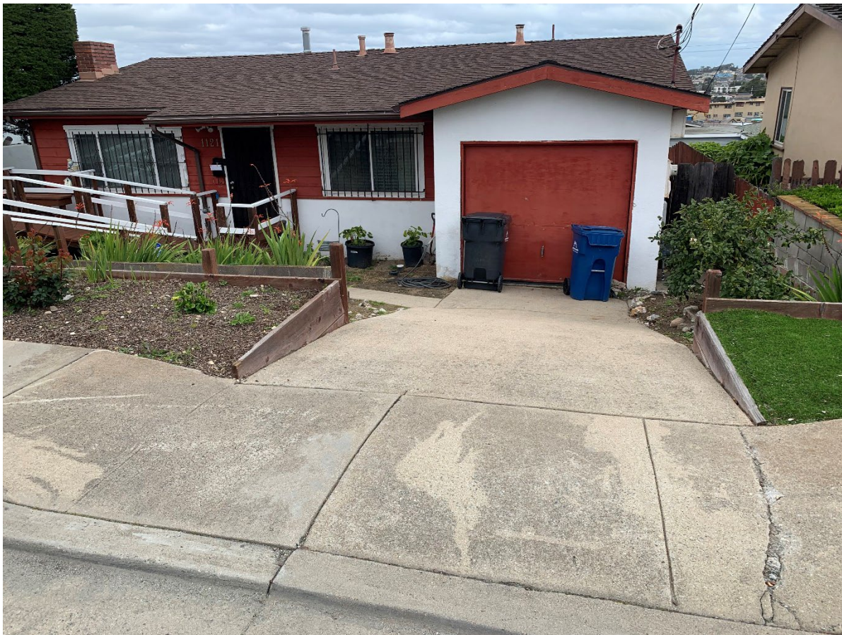
Applicant's driveway and garage
