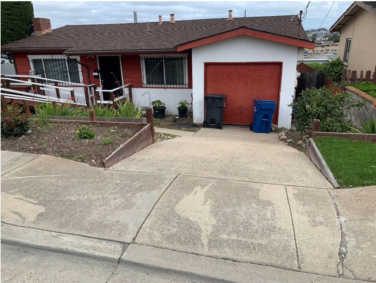
Applicant's driveway and garage
