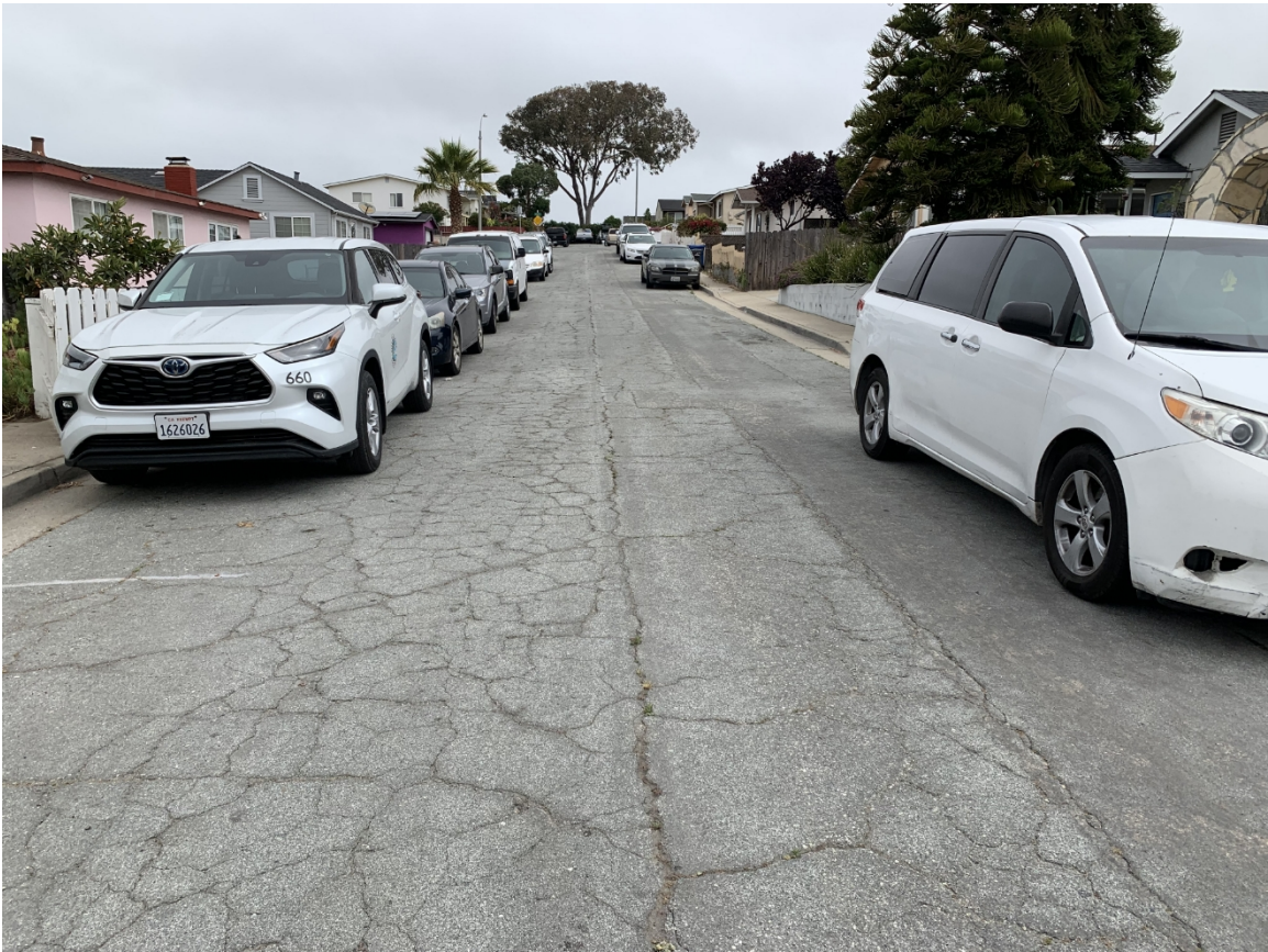
View to the north
