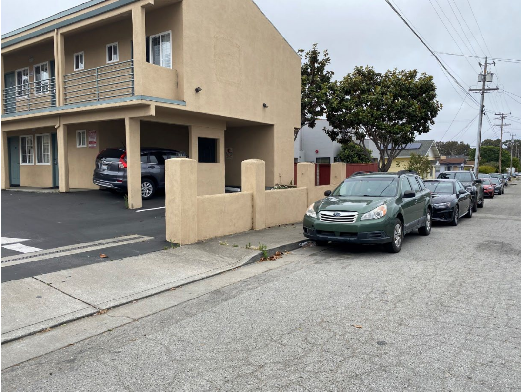
Francis Avenue looking west
