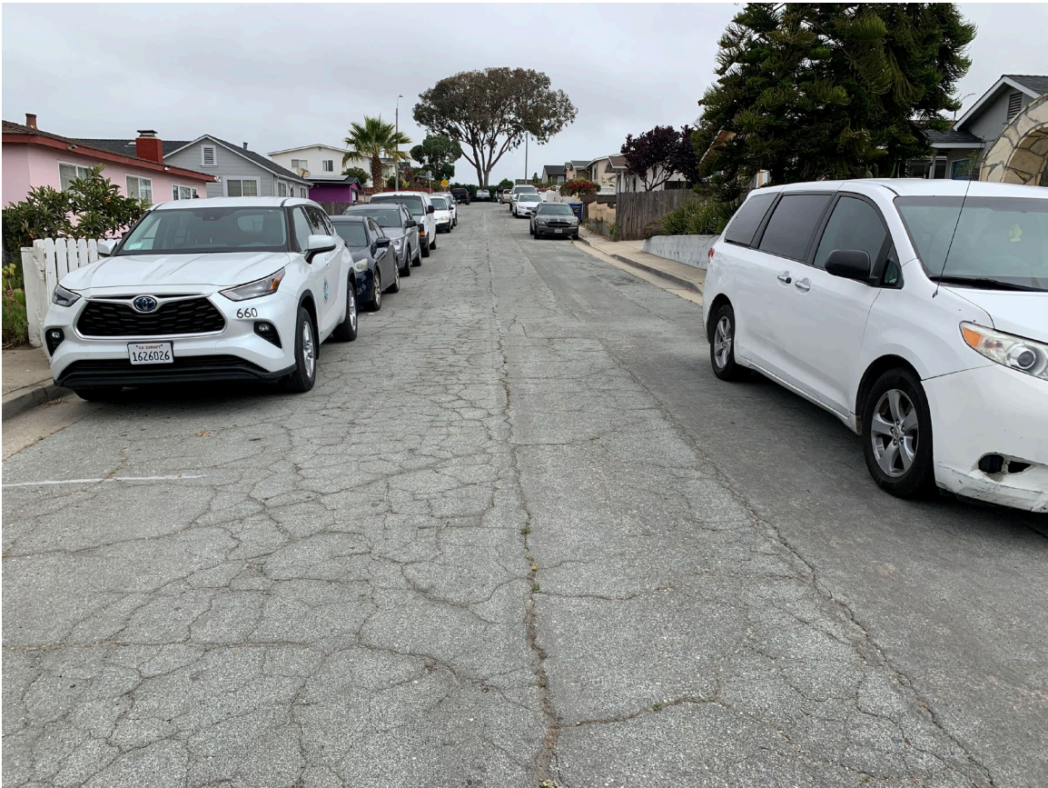
View to the north
