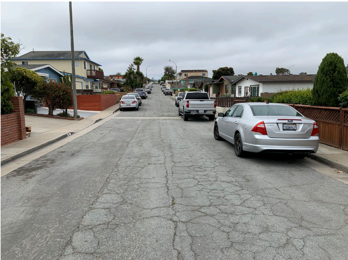
View to the south
