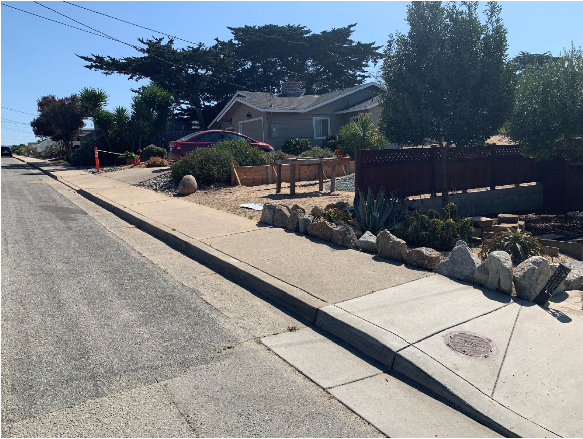
Fence in safety visibility area, less than 48" in height. Code compliant.
