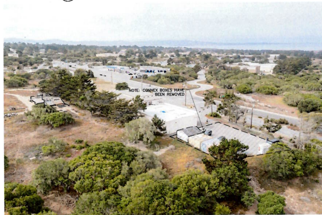
C FIRE STATION NORTHEAST SIDE; SOUTHWEST FACING VIEW C-01 NOT TO SCALE
