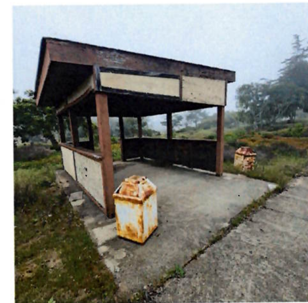
C SOUTHWEST STRUCTURE CLOSEUP C-25 SCALE: NTS
