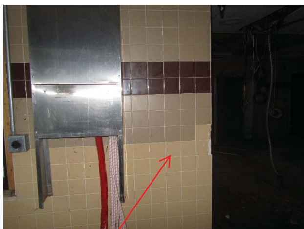
Lead-Based Ceramic Tile
