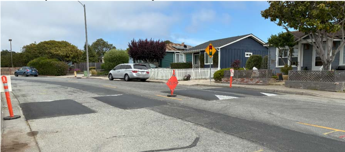
Lower Hilby west of Santa Theresa – Speed Cushion Installation
