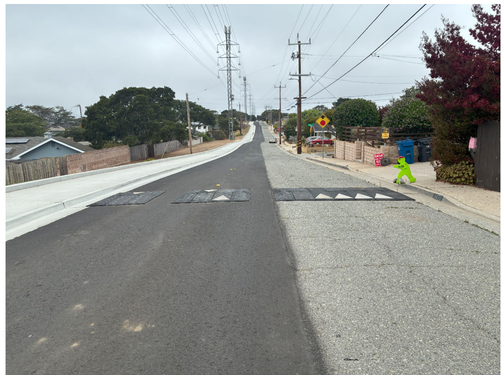
Existing Speed Cushions between 1463 & 1471 Plumas Ave looking westbound towards Waring Street
