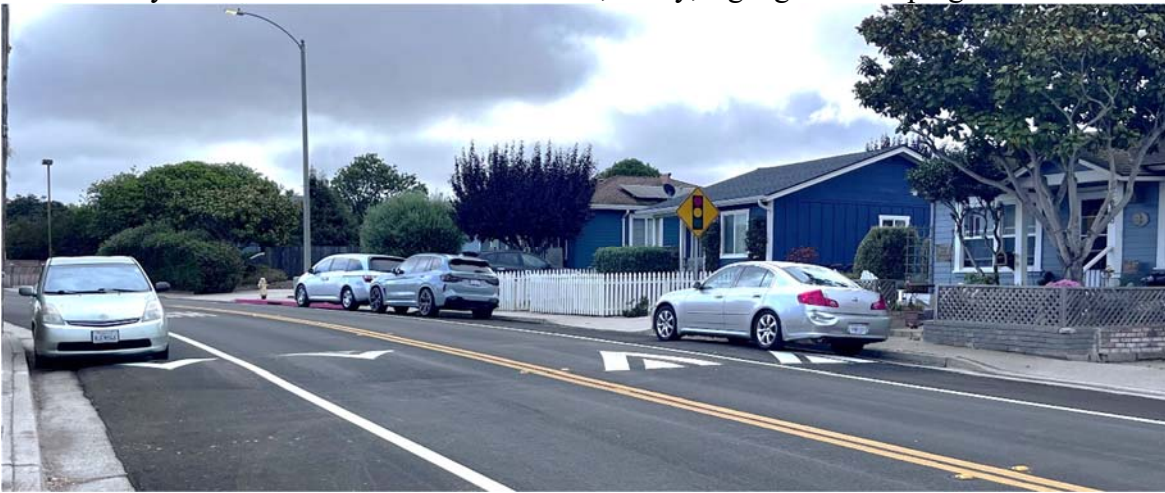
Lower Hilby west of Santa Theresa – cushions, slurry, signage and striping
