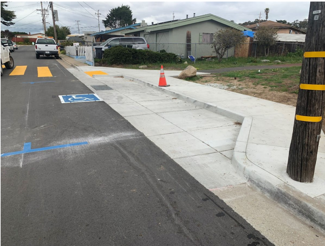
Example of recessed ADA compliant parking space being constructed on Lincoln St.
