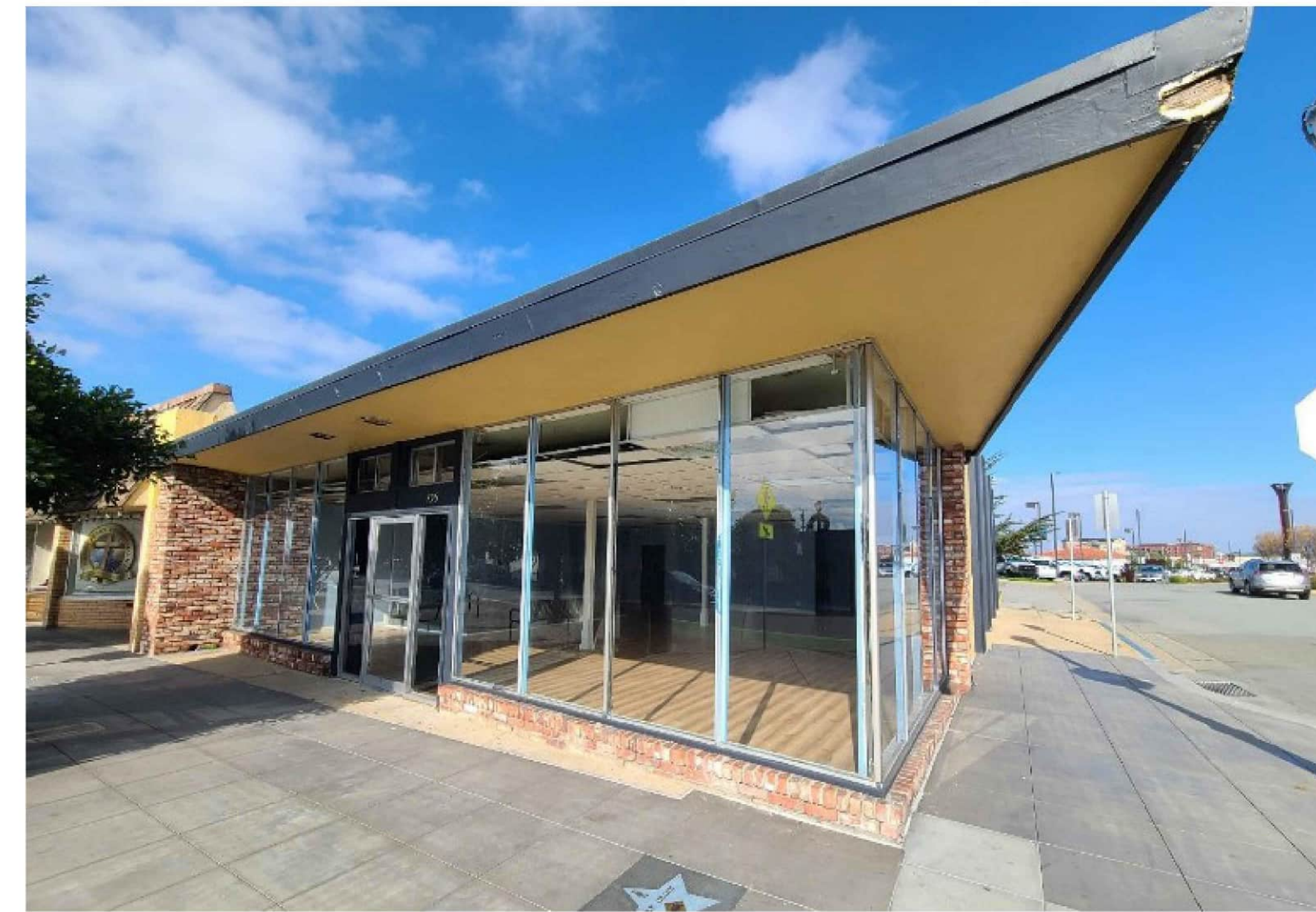
BROADWAY/ STREET VIEW OF EXISTING (NO CHANGES)
