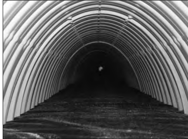
Looking down the Isolator Row
