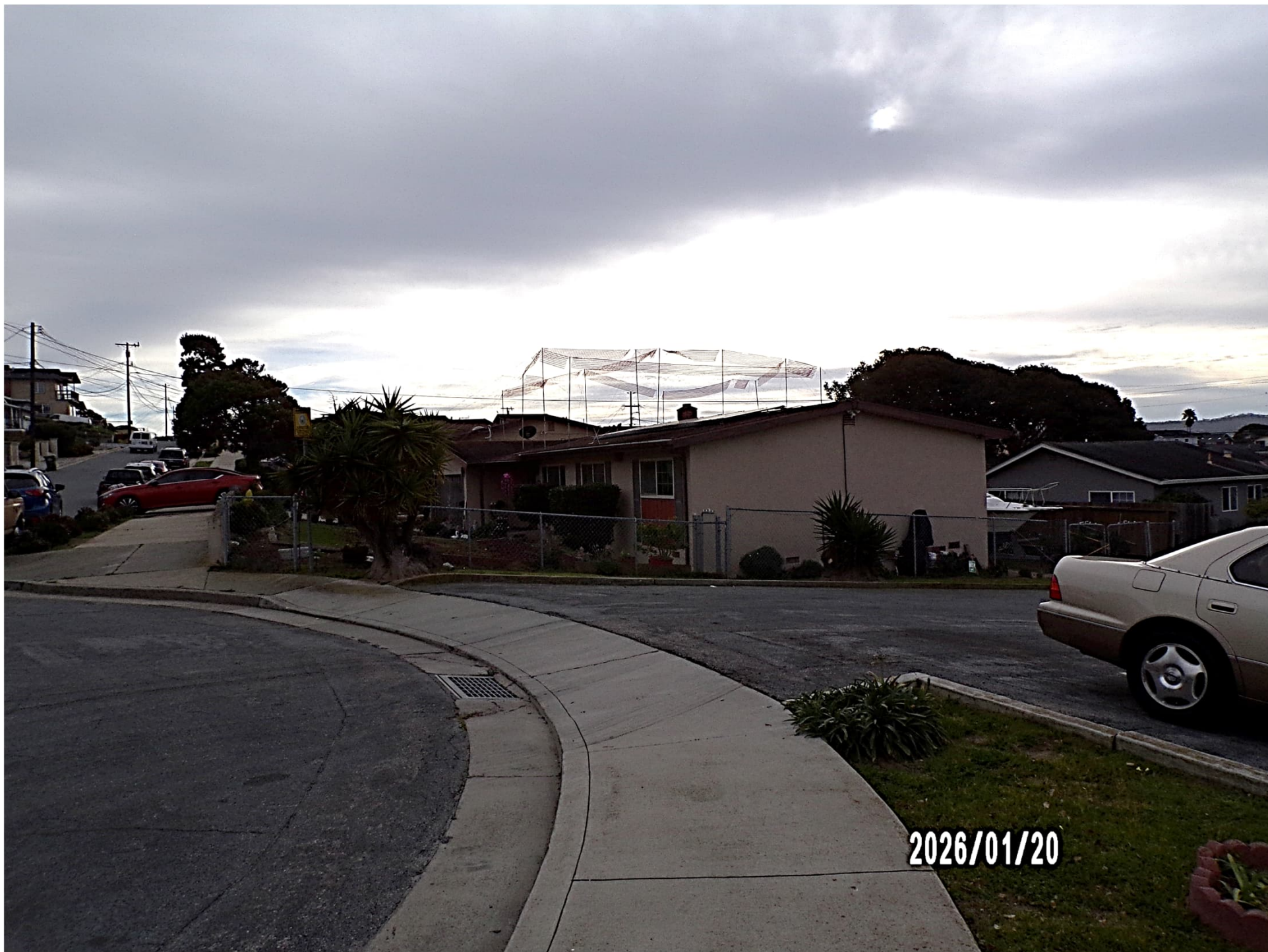
Staking and flagging shown from the parking lot directly to the north. The downward slope from east to west is visible.
