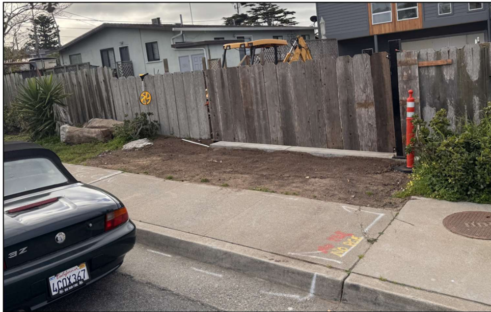
Existing Conditions at the Proposed Driveway Approach Location.
