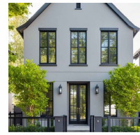
EXTERIOR STUCCO PAINT: (N) EXTERIOR STUCCO: SAKREITE SCRATCH & BROWN W/ BEHR PREMIUM #MS-66 NEW ENGLAND GRAY FINISH.
