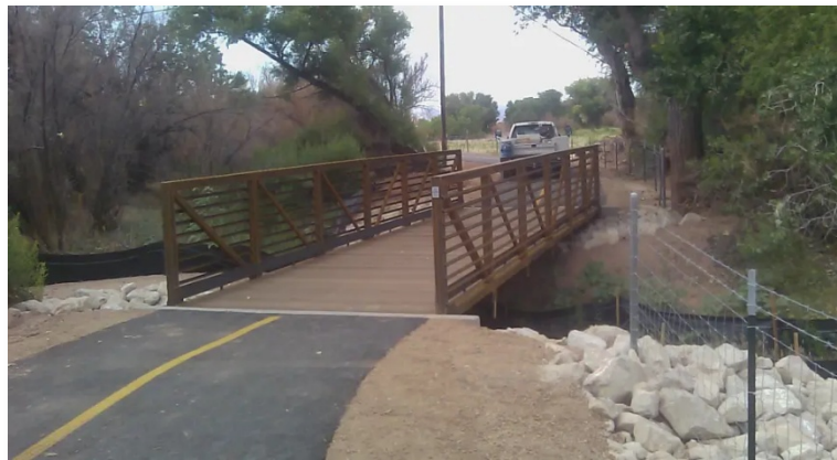
Example Connector Bridge with Timber Deck
