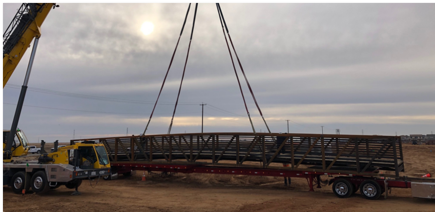
Example Bridge Assembly with Crane
