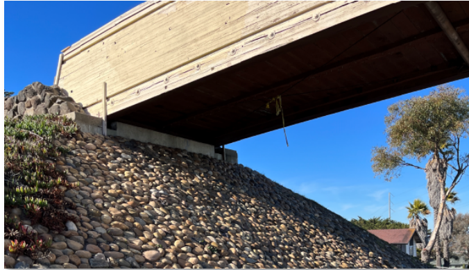
Existing Slope Protection
