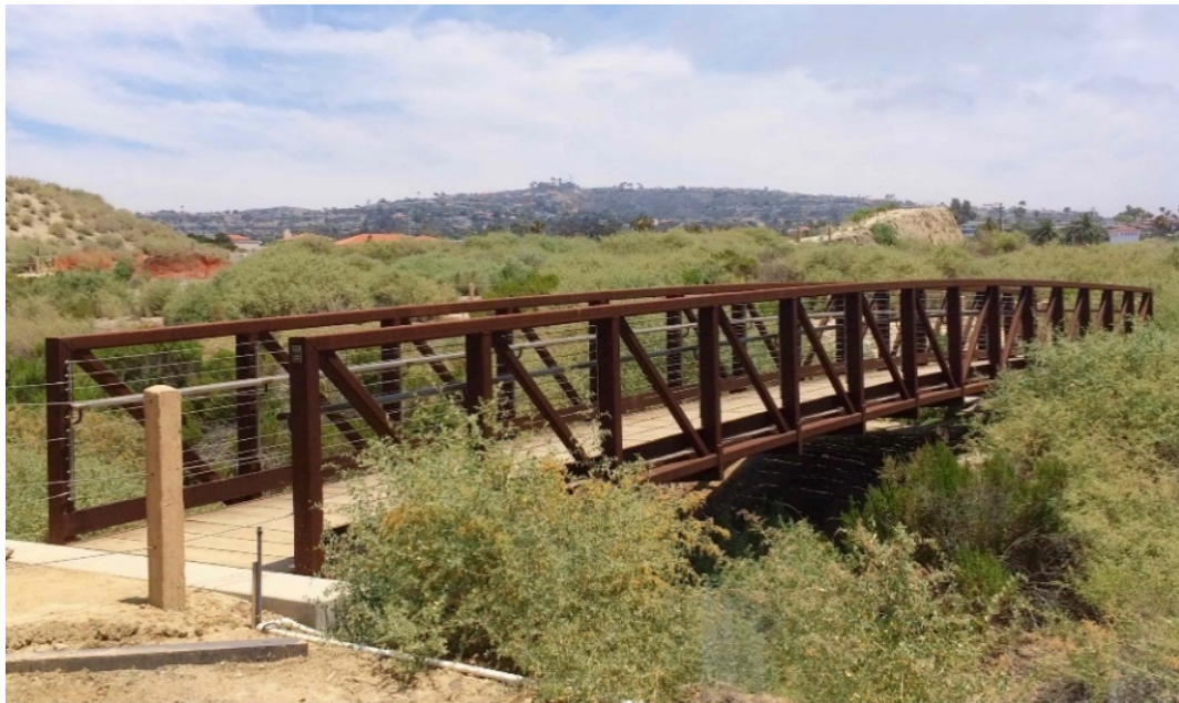
Example Prefabricated Truss Bridge
