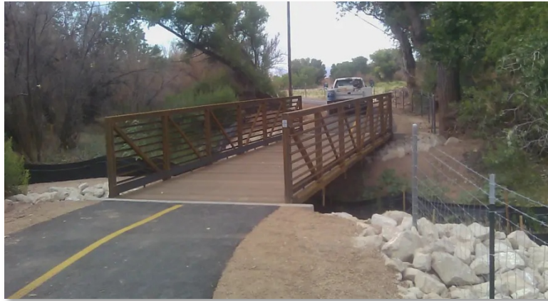
Example Connector Bridge with Timber Deck
