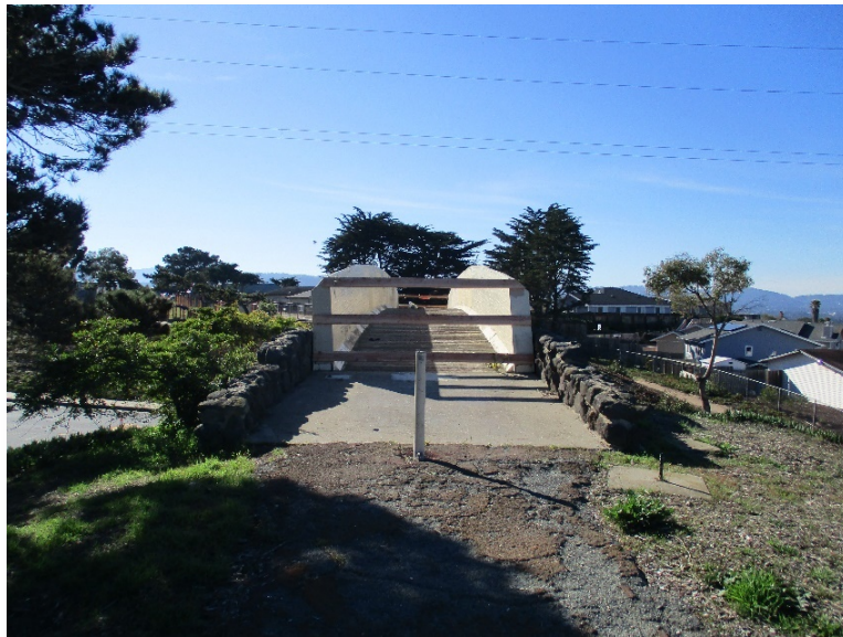
Existing Bridge Closure
